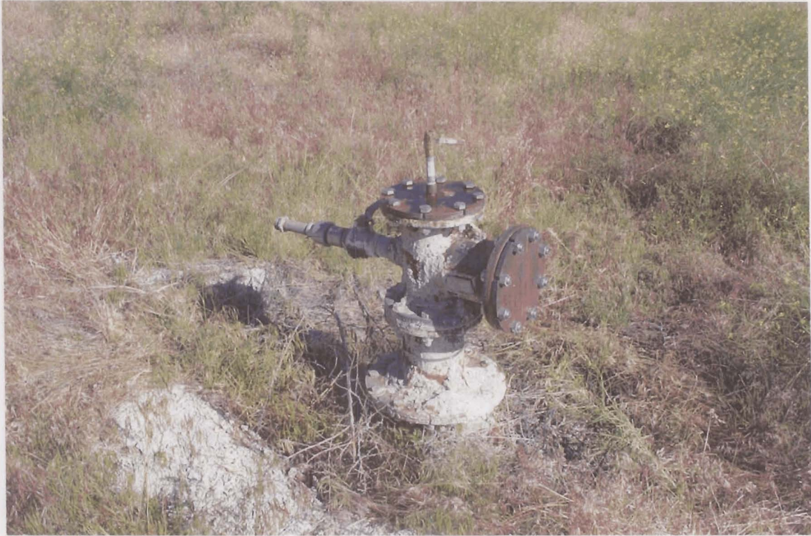
Existing Geothermal Well On Lot 2 Oregon Trail Subdiv. App For Permit 47-17127 By J E Stanton 6-4-04
