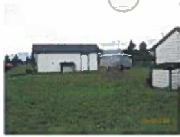
BOOSTER PUMP HOUSE.JPG
