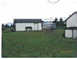
BOOSTER PUMP HOUSE.JPG
