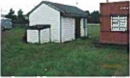
PUMP HOUSE WELL #1.JPG
