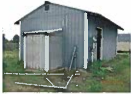
PUMP HOUSE WELL #2.JPG
