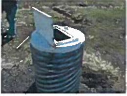
POINT OF DIVERSION 1
