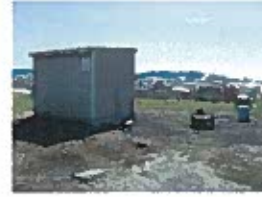
PUMP HOUSE AND POINT OF DIVERSION 1
