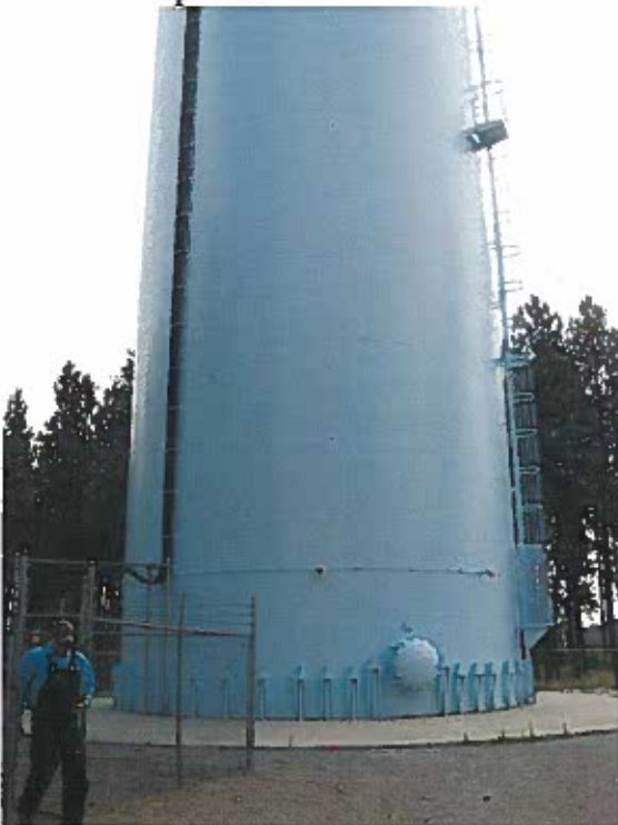
PF Wells 5 & 7 Reservoir
