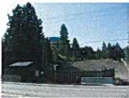
3rd AVE Lift Station and Reservoir.JPG
