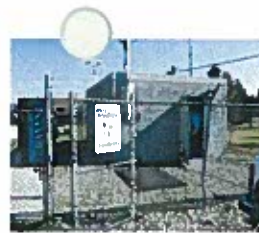
PF Well 4 Exterior.JPG
