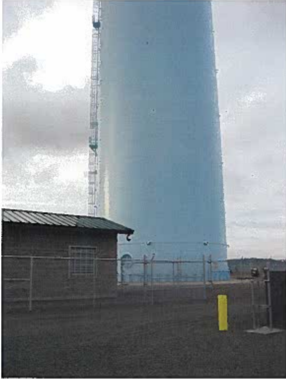
Well 9 and Reservoir
