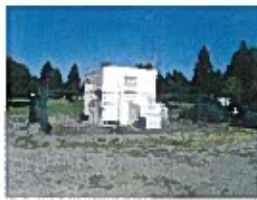
PF Well 3 Exterior.JPG
