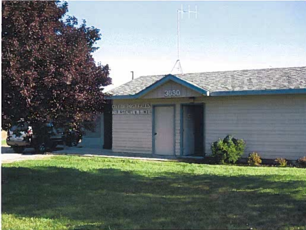
95-8768 Well House POD
