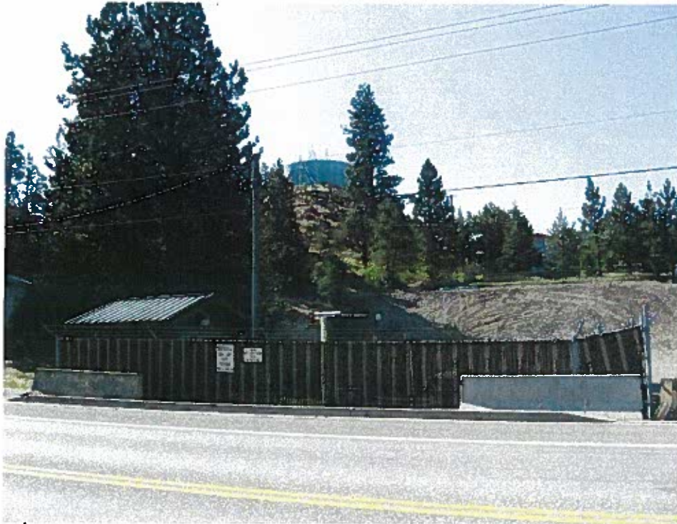
3 rd AVE Lift Station and Reservoir
