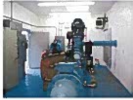
PF Well 5 Interior.JPG
