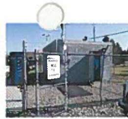
PF Well 4 Exterior.JPG
