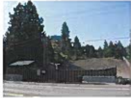
3rd AVE Lift Station and Reservoir.JPG
