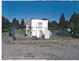
PF Well 3 Exterior.JPG
