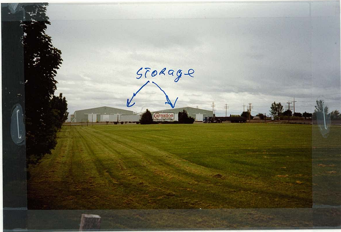
FRONT View OF the Facility.
