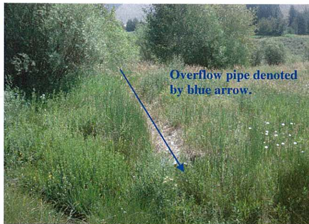
- Point where overflow pipe discharges. Small stream visible in bottom left of picture is water from pond spill way.
