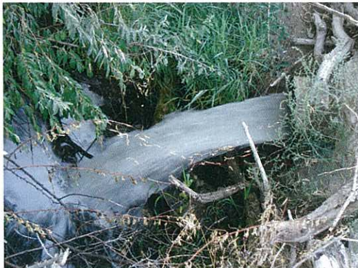
Below: Close ups of the outlet discharge and spillway.
