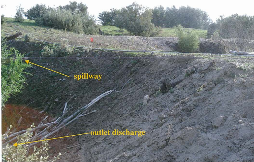
Above: View of the dam. Spillway is the culvert in the upper left and the outlet discharge is in the bottom left.
