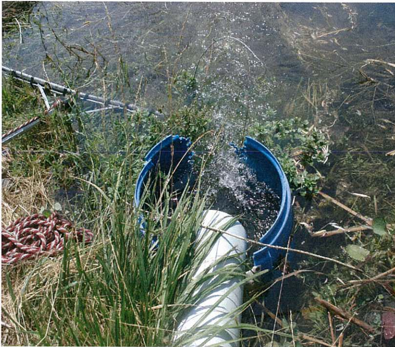
- Point where waste water enters pond thru underground pipeline.
