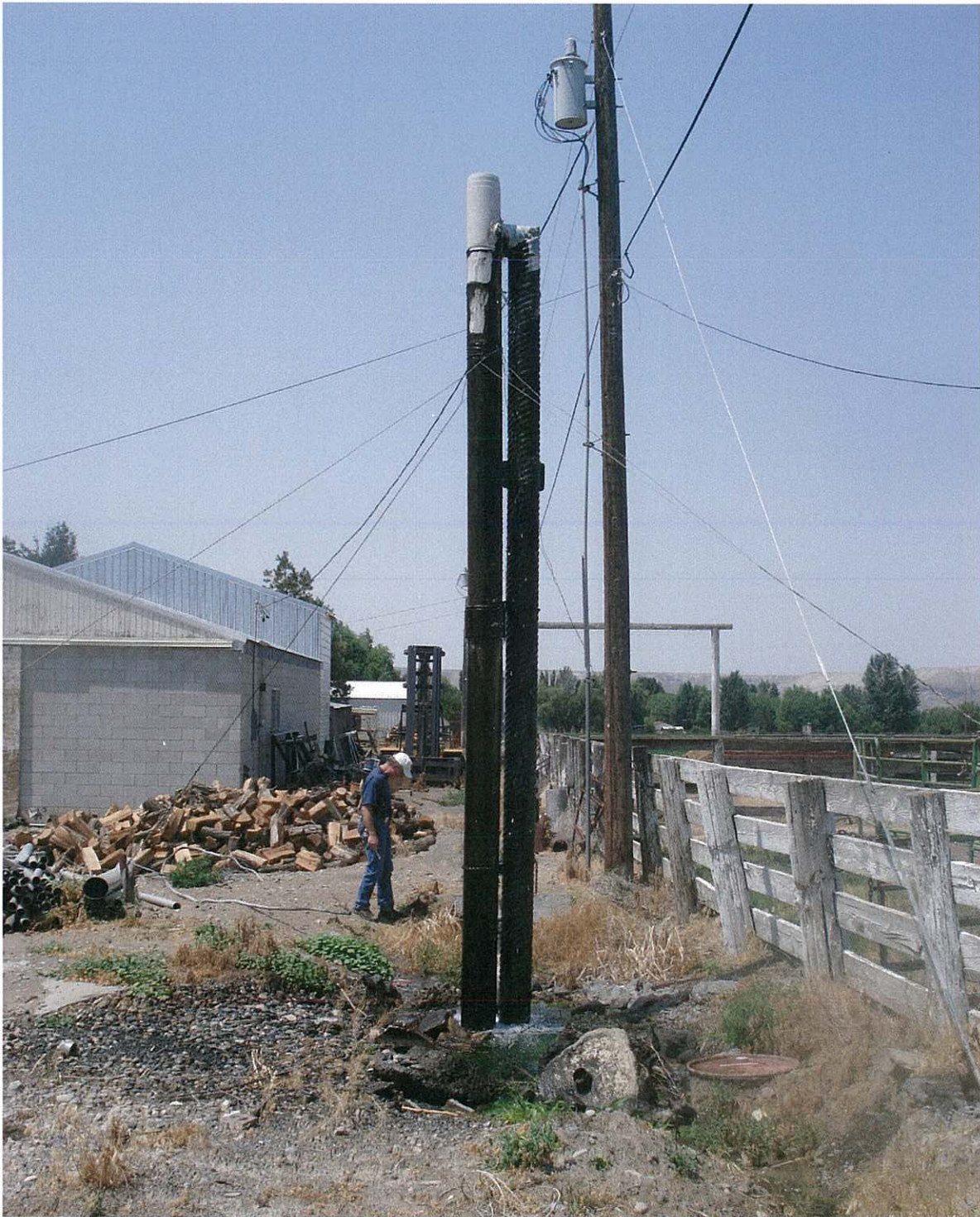
- BIG SPRINGS OVER FLOW PIPE
