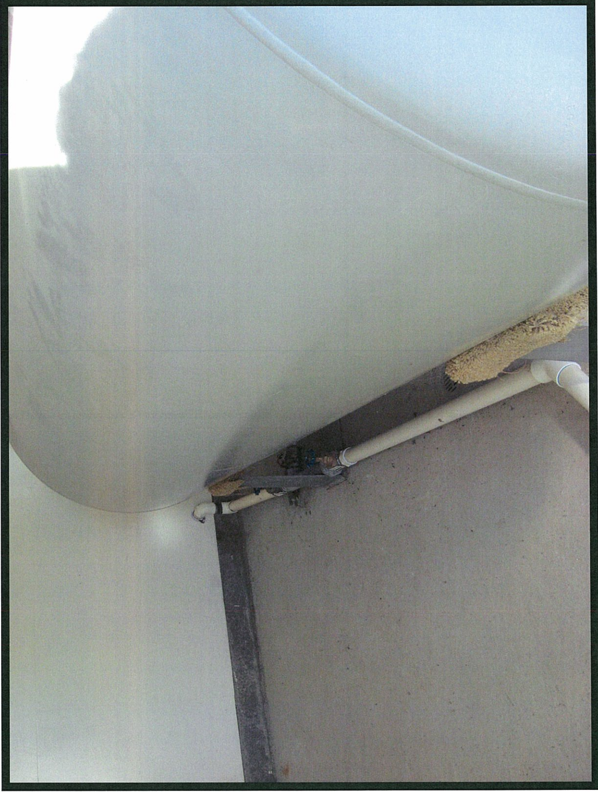
Friends Well Storage Tank
