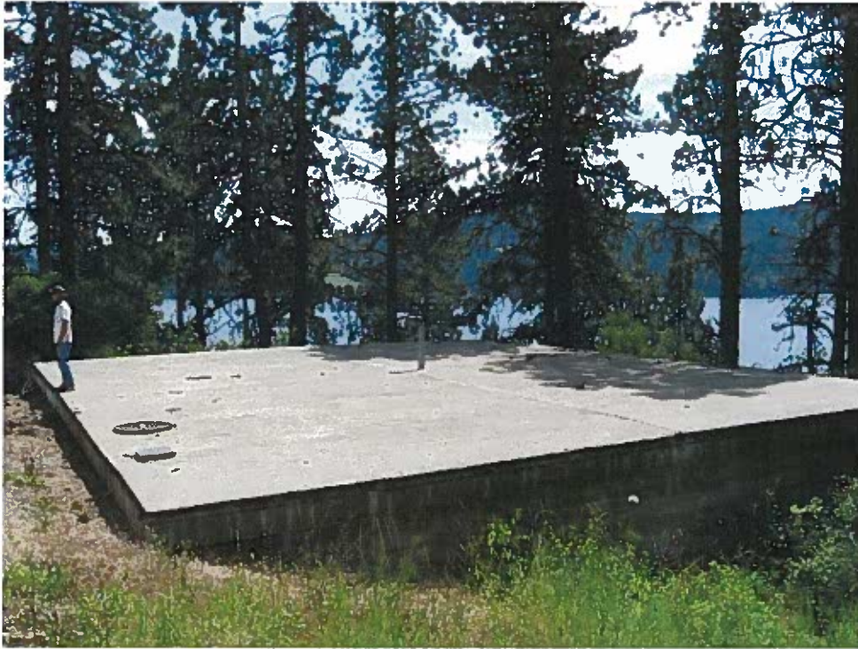
94-7383 Low Reservoir & City Employee
