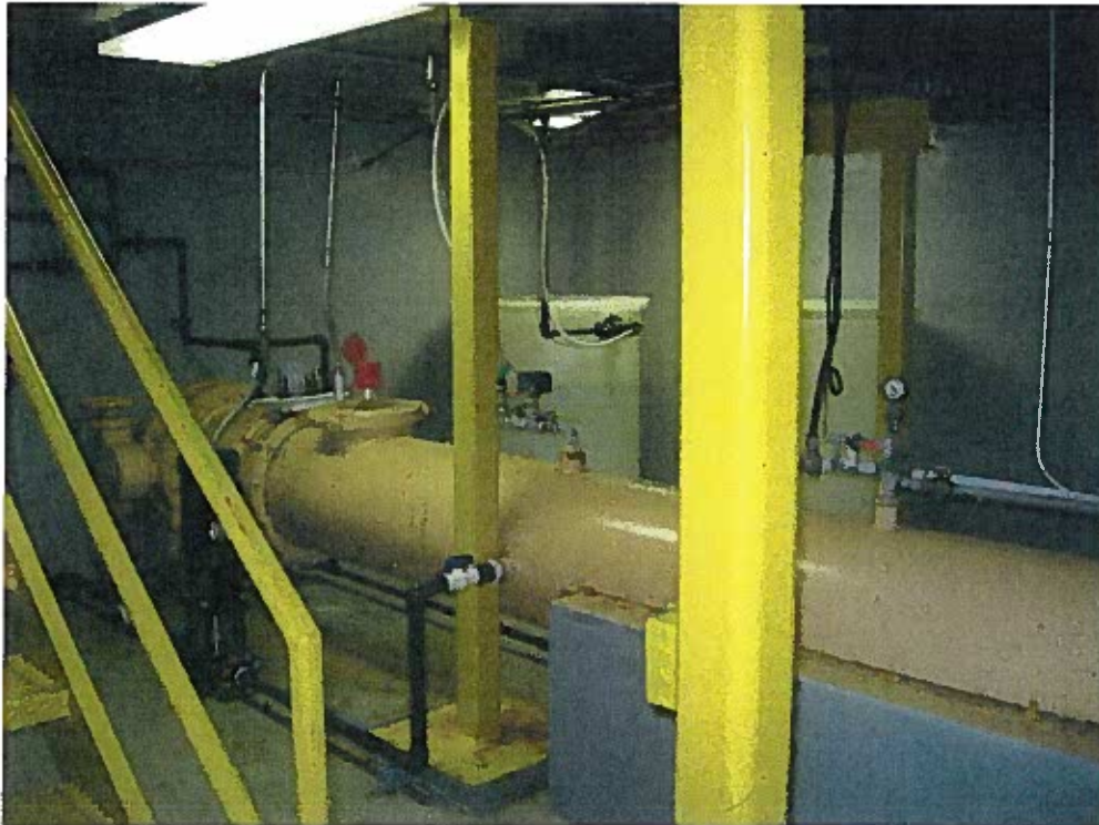
Miles AVE Well Site Control BLDG
