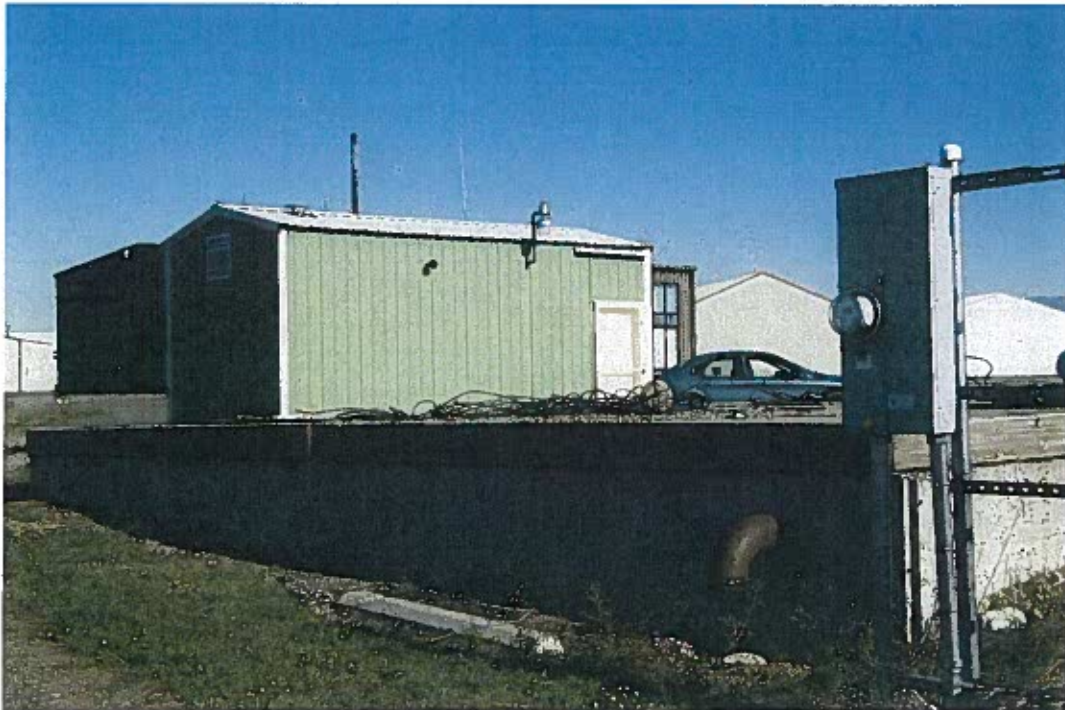
Airport Well 1, POU & Unused Reservoir
