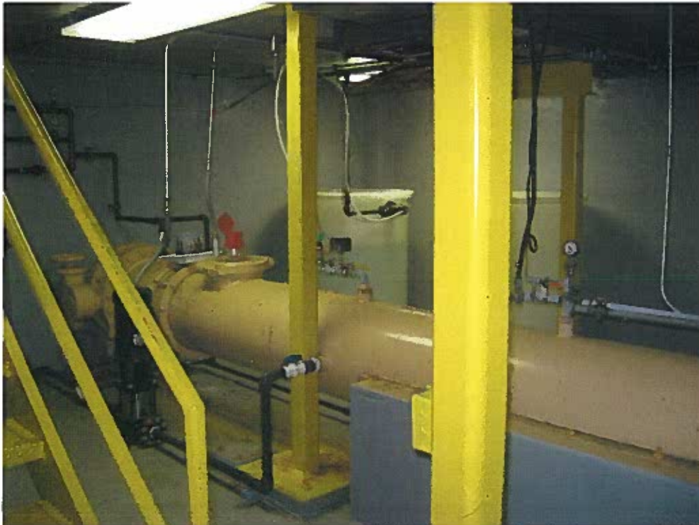
Miles AVE Well Site Control BLDG
