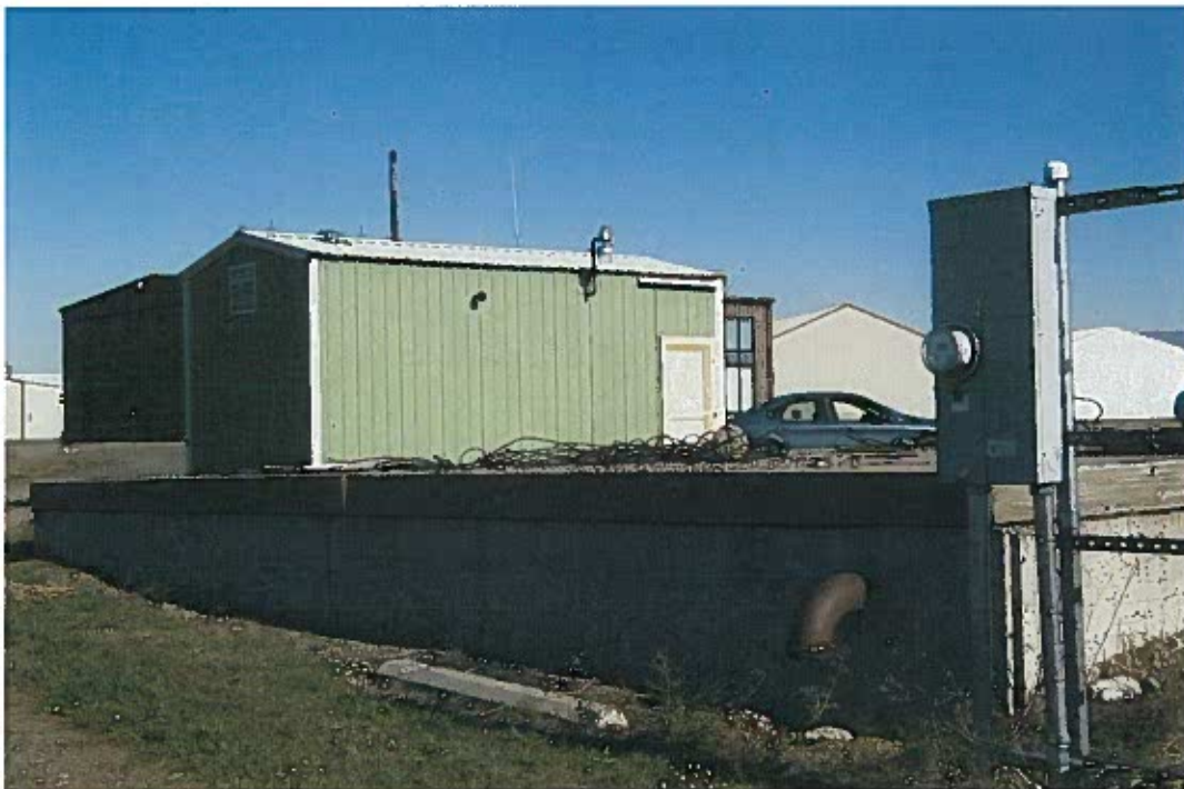
Airport Well 1, POU & Unused Reservoir
