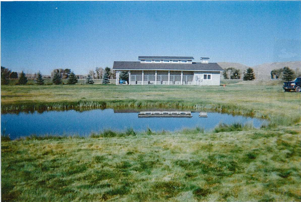
Commercial building. Picture taken facing west.
