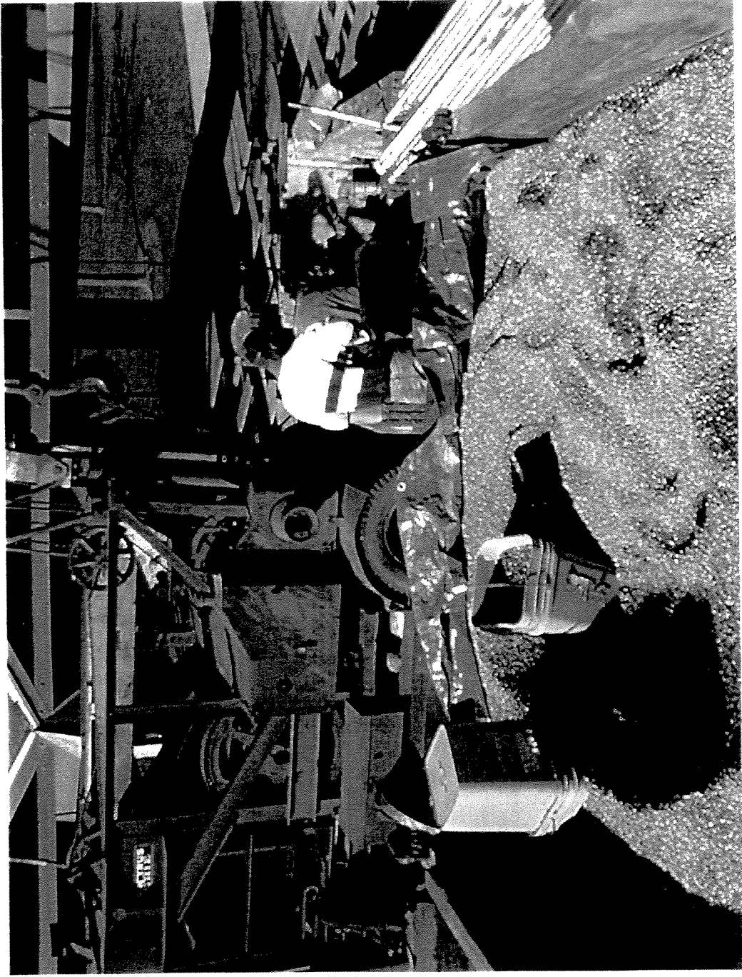
Gravel Pack Material in Dump Truck (pipe to the right is tremie pipe)
