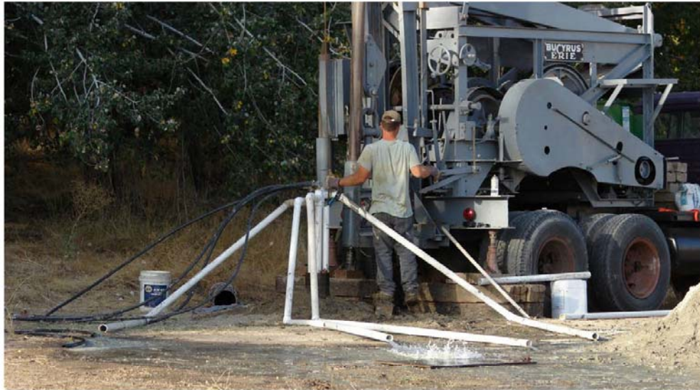
Figure 17. Well Development, Wellhead Shelter, and Small-Diameter Wells within a Single Borehole
