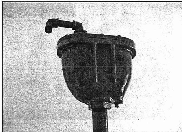
Fig. 12 – air relief valve
