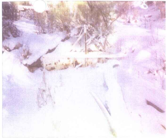
B Our Clark Ditch headgate 1-5-07
