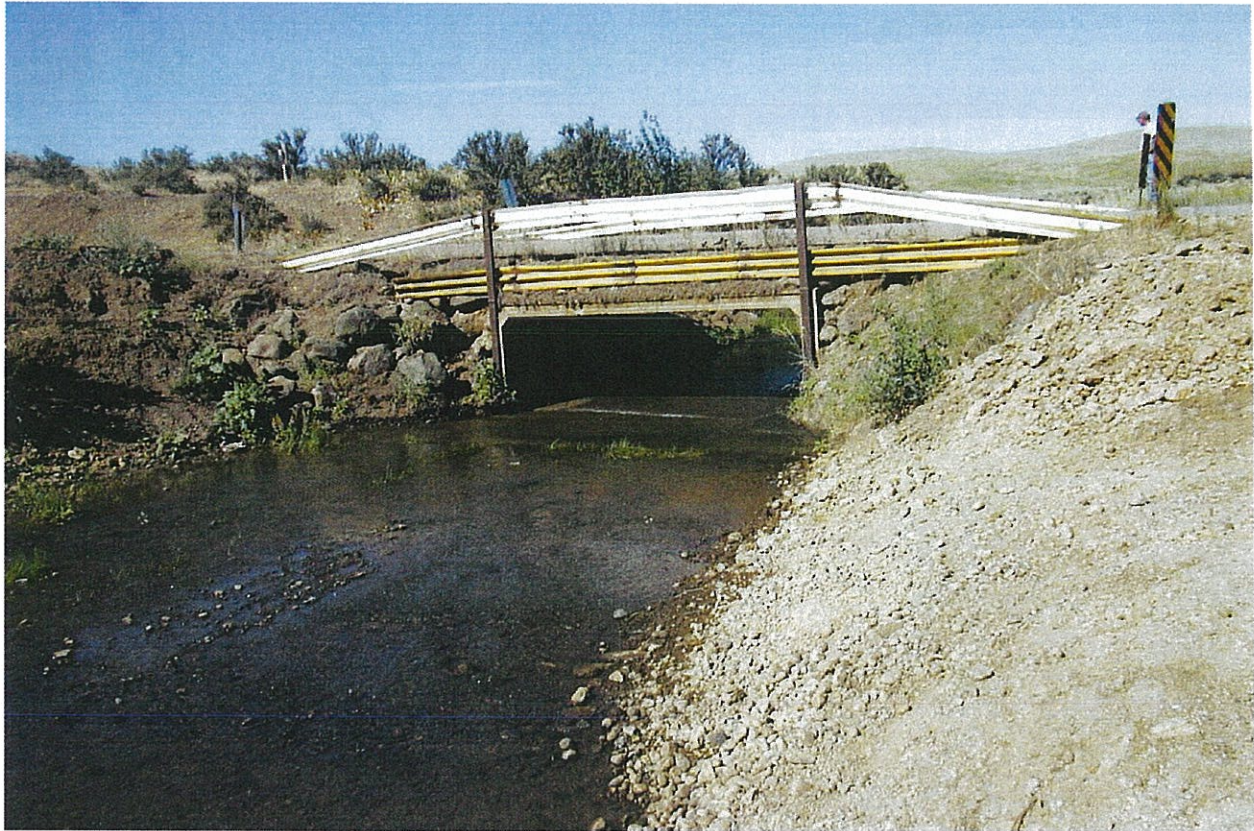
Photo #2: Spillway channel looking downstream to road bridge, loose fill and rock have been removed from the channel, significant improvement.
