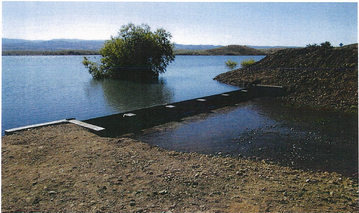
Photo #1: Overview of the new structure with flashboards, good.
