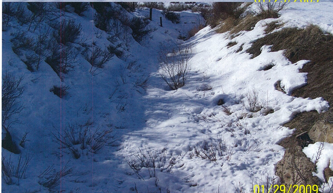
west side spillway dirt ditch (left abutment)
