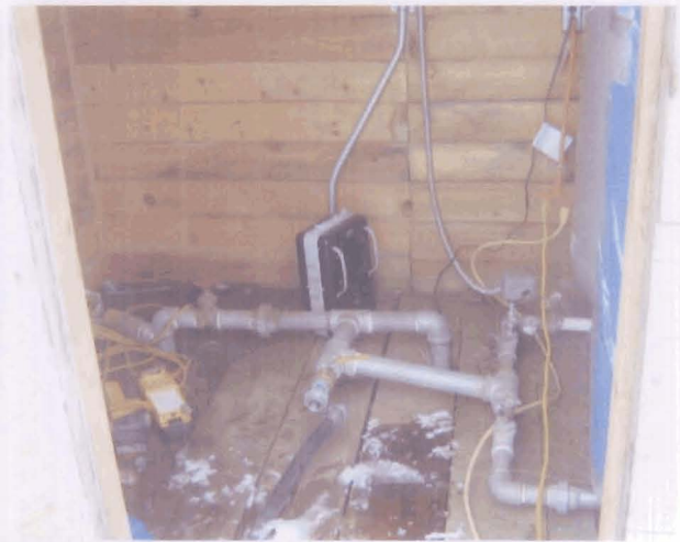
Piping & pressure tanks inside well house
