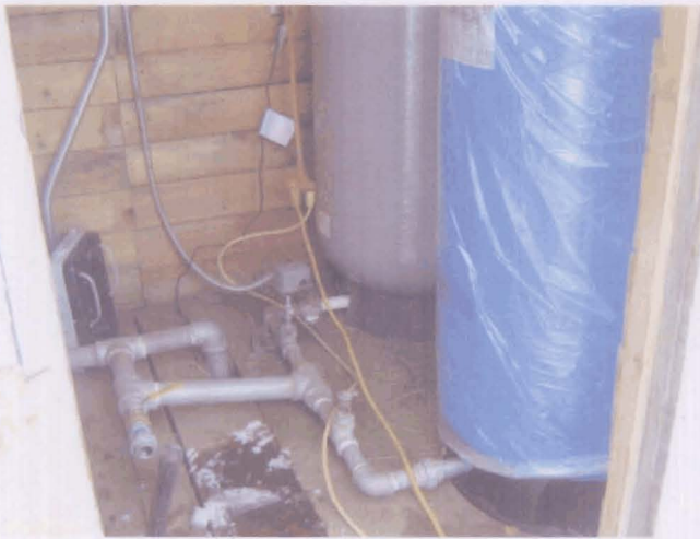
Piping & pressure tanks inside well house
