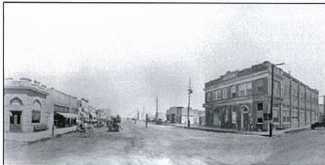
Main & Little 1921 – Looking North
