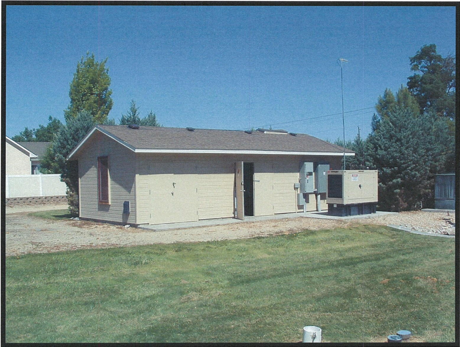
Well and Pump House
