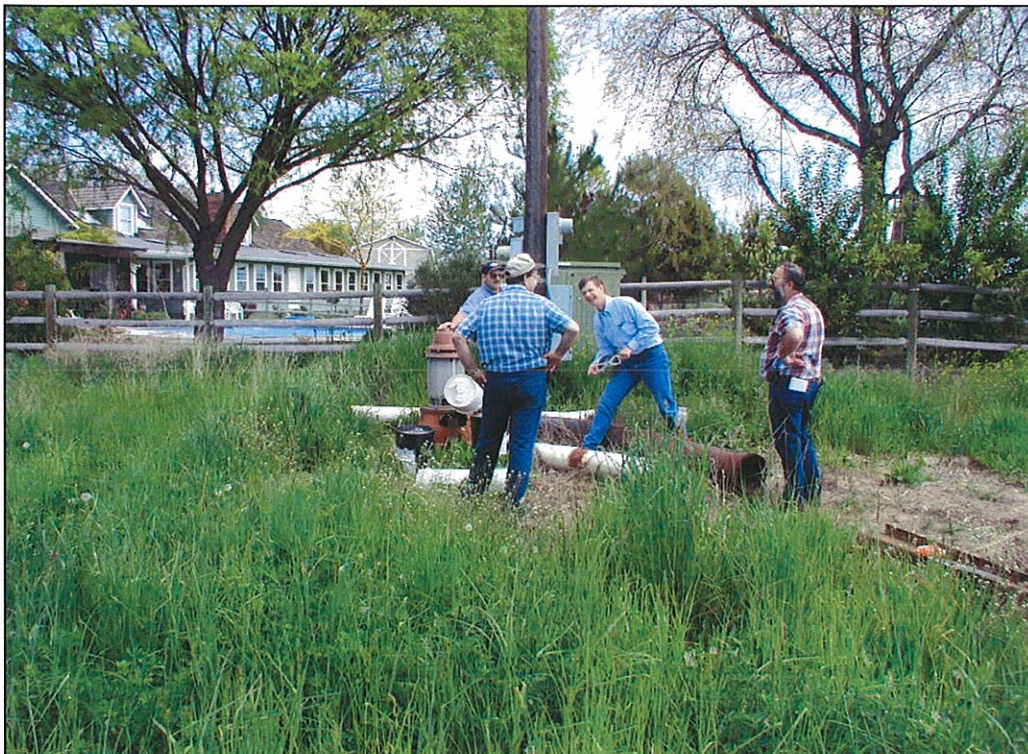
Looking East at well head. Big irrigation well, 5/13/03, 14:14 hrs, photo by Chris Duncan - Holladay Engineering Company. Photo 9
