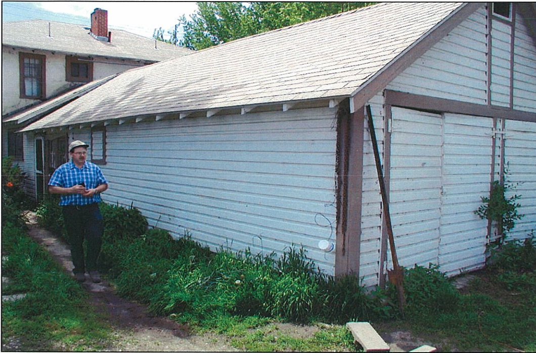
Looking S.W. at building with well. Dairy / House Well, 5/13/03, 13:40 hrs, photo by Chris Duncan - Holladay Engineering Company. Photo 3
