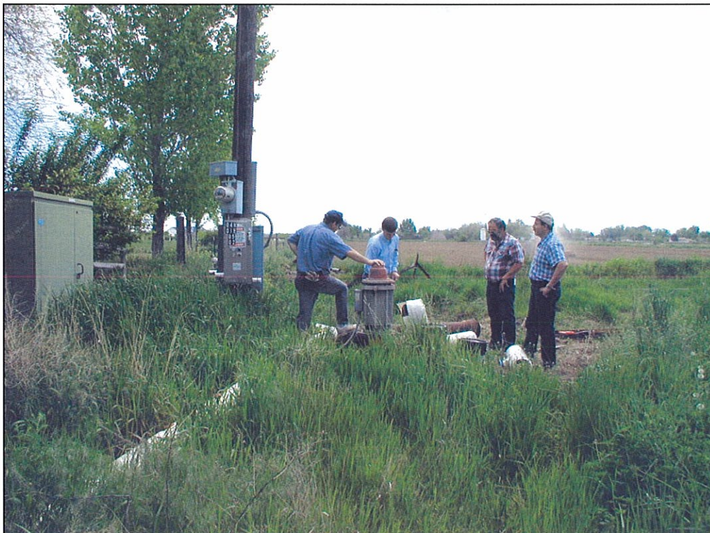
Looking South at well head. Big irrigation well. 5/13/03, 14:14 hrs, photo by Chris Duncan - Holladay Engineering Company. Photo 10
