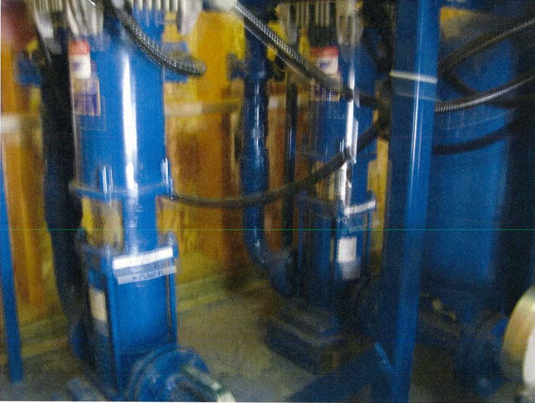
Photo 9 8 and 10 9: Diversion works that pump the water from the 10,000 gallon holding tank to the park and buildings.
