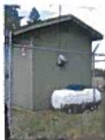
95-8057 Hidden Valley Transfer Station.JPG
