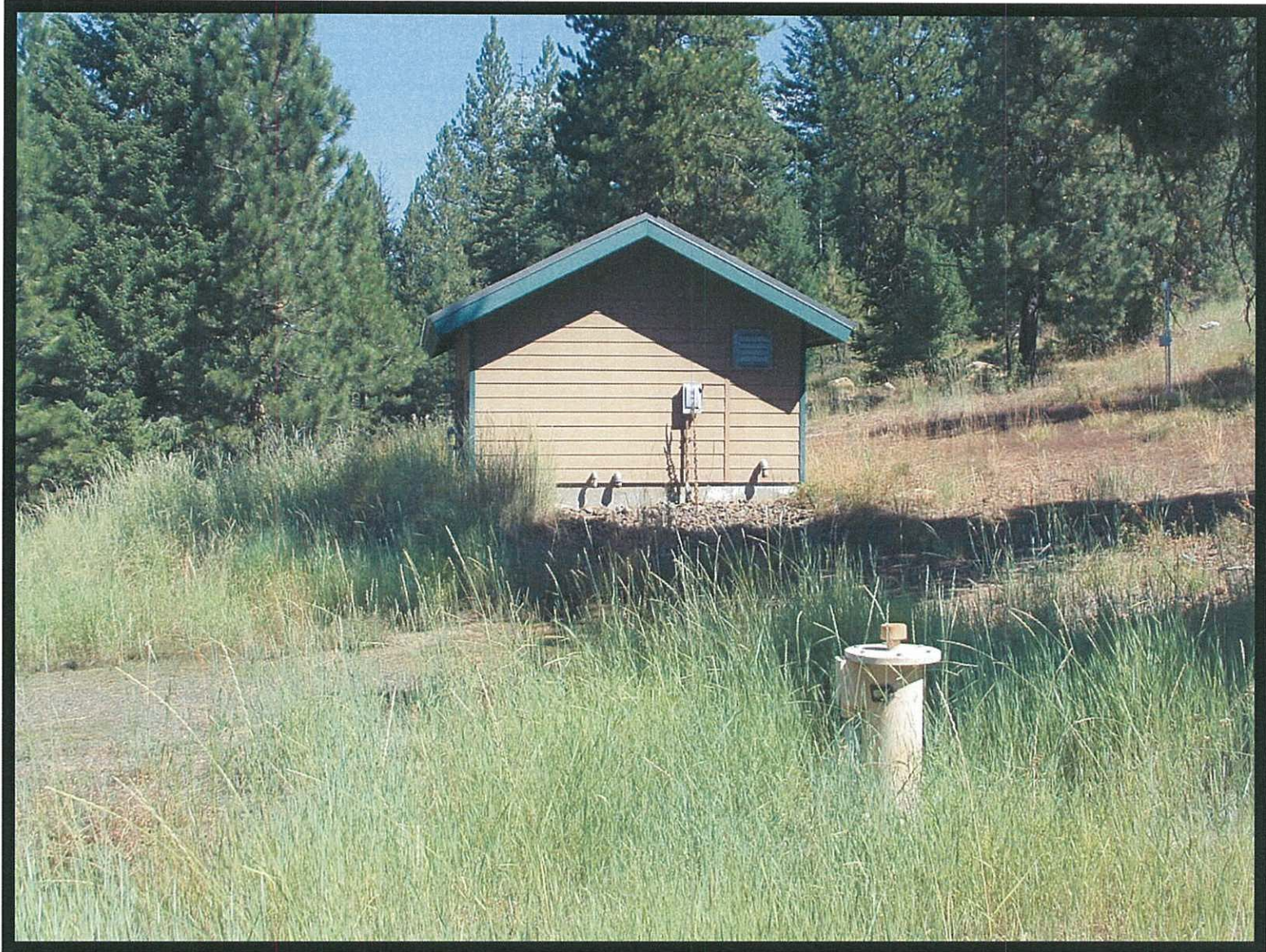
South Well and Well House
