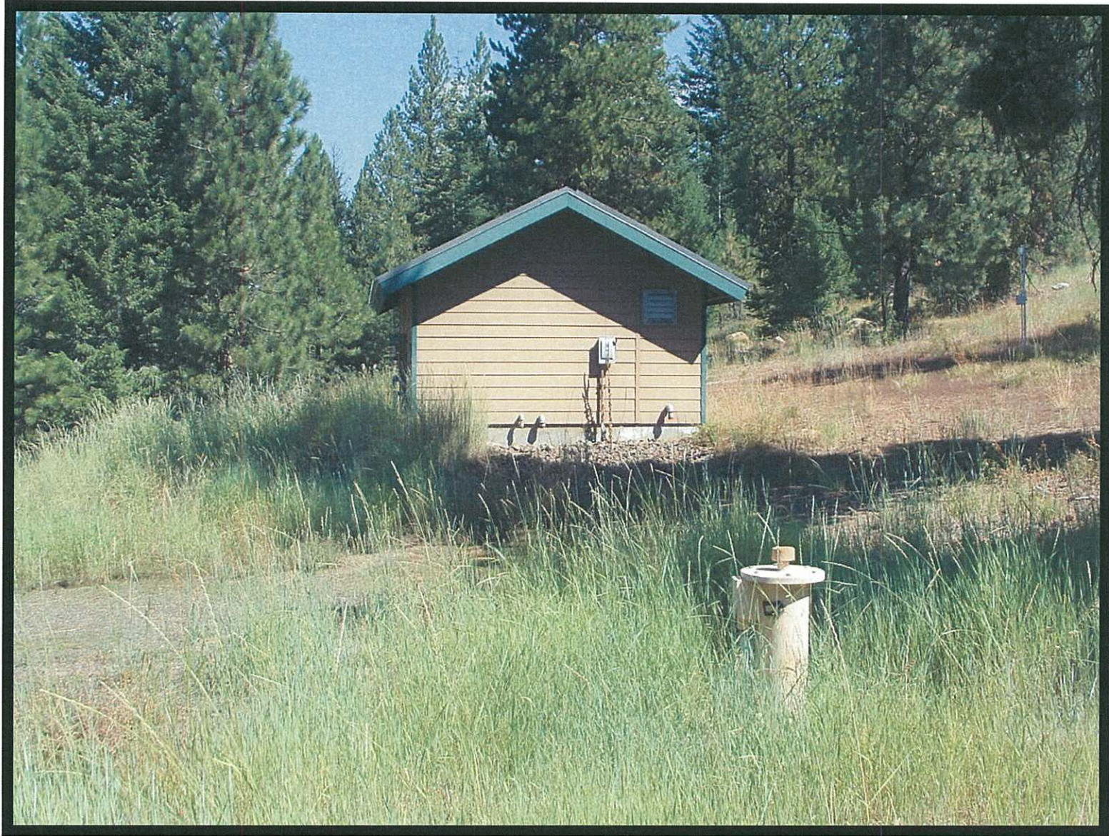
South Well and Well House
