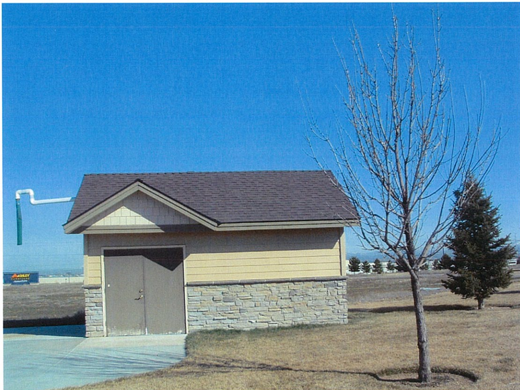
Well house building.
