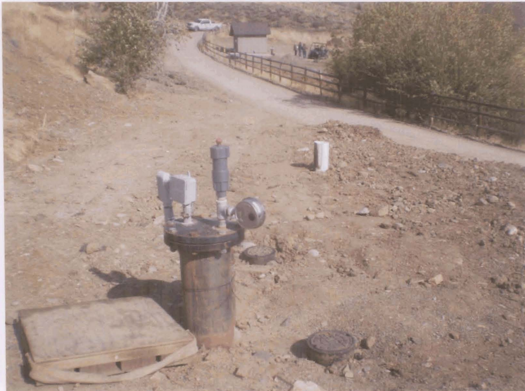
Well #11, looking north
