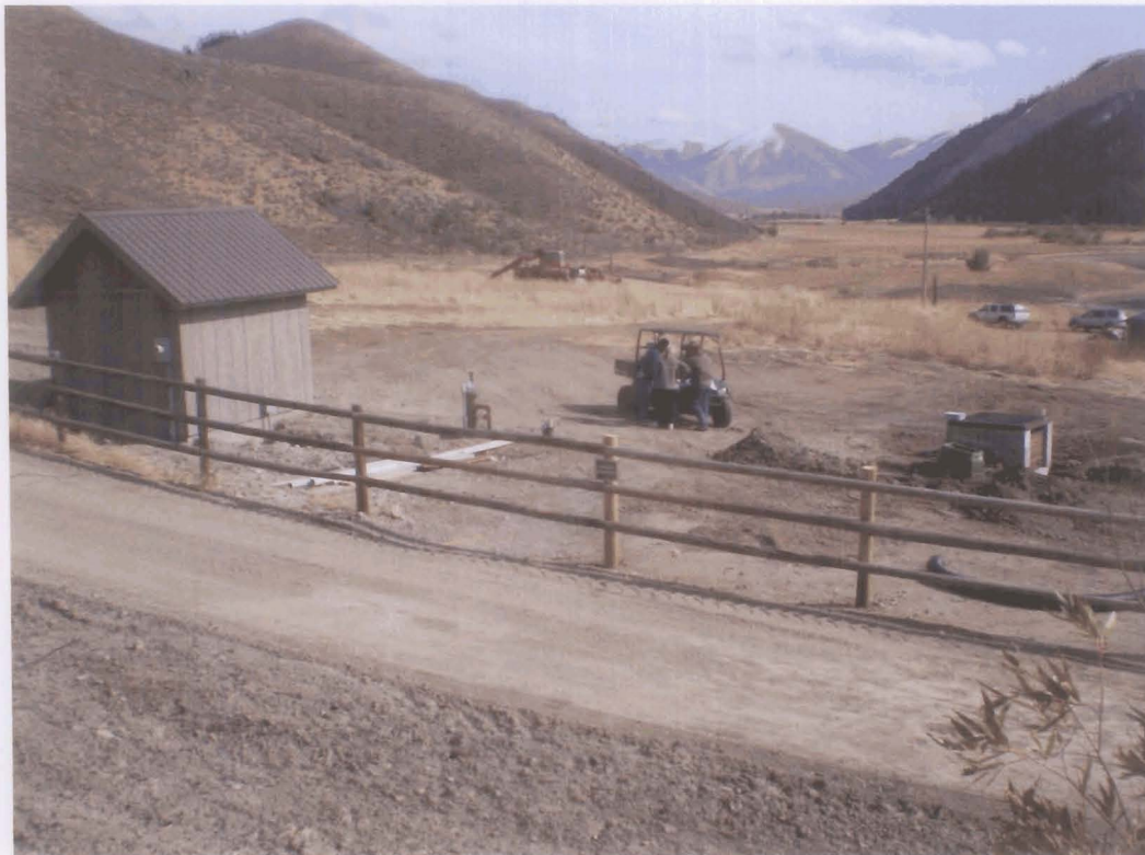
Control house (left), Well #75-1 (left of center), and collection box (right)
