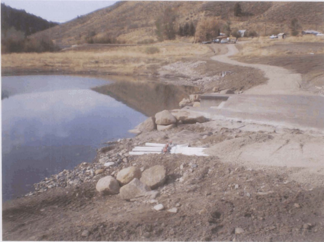
Pond / spa, terrace, path, and return pipes (looking west)
