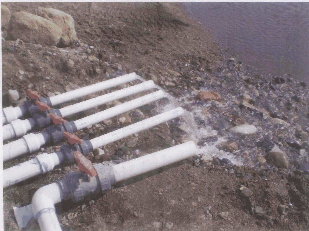
Return to pond for snowmelting Zones 2, 4A, 4B, 4C
