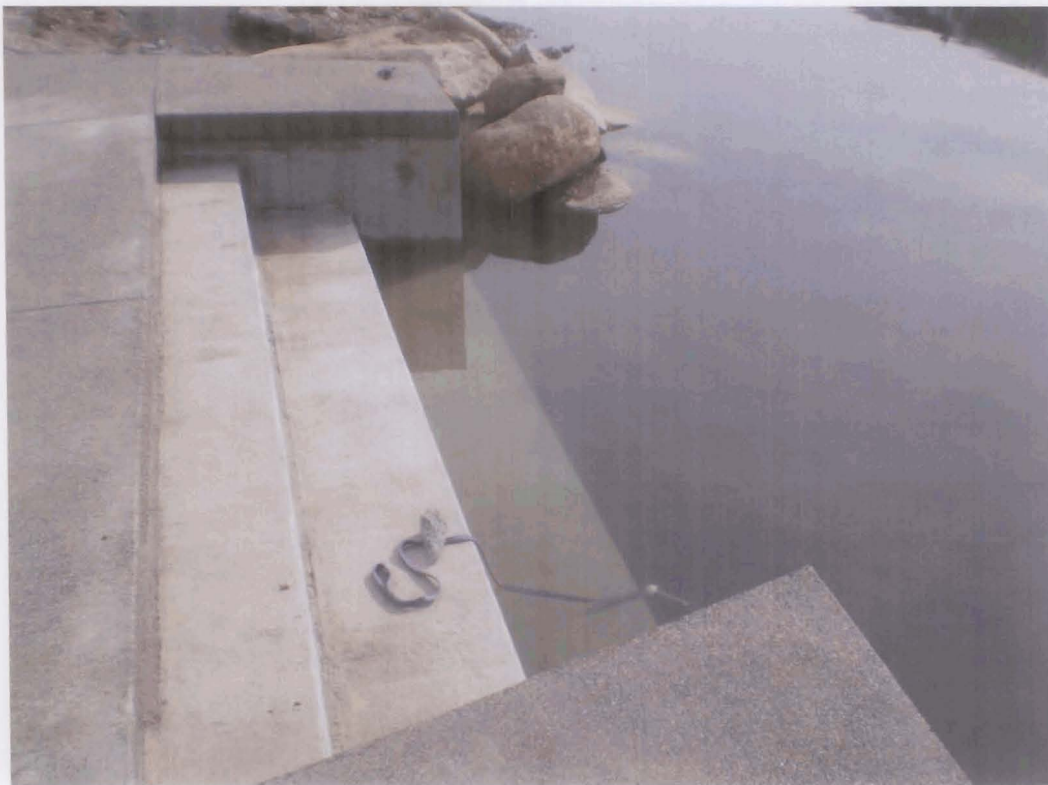
Terrace & steps – access to pond / spa
