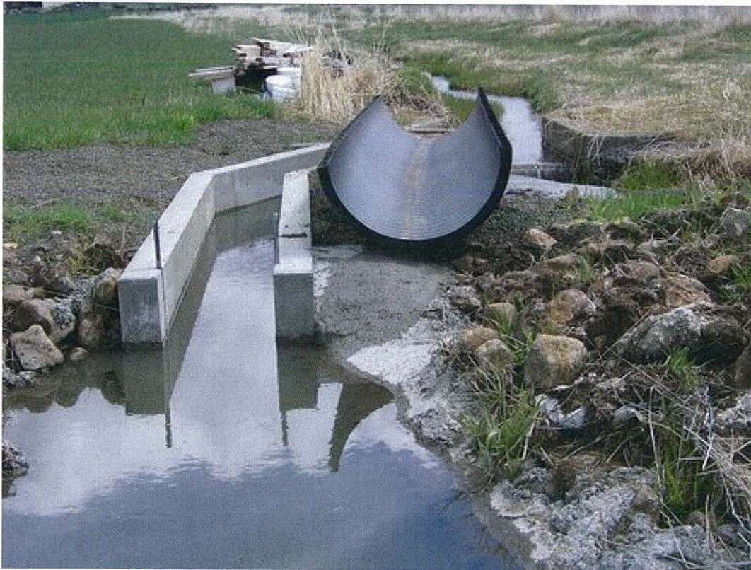
Downstream of diversion in conveyance channel to Tolo Lake looking upstream at the point of diversion, Spring/Summer 2009. Leaky basalt caissons (previous picture) have been replaced with concrete walls. Conveyance channel has been lined with cement downstream of end of diversion.
