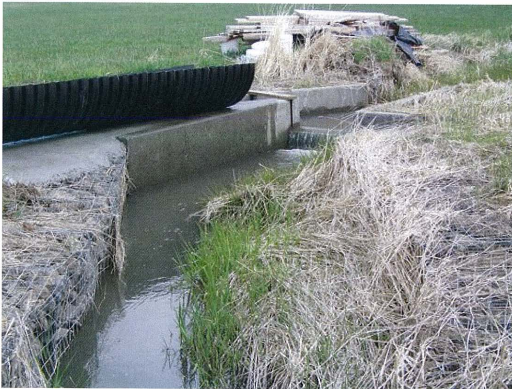
Downstream of diversion in Techler Creek channel looking upstream at the point of diversion, Spring/Summer 2009.
