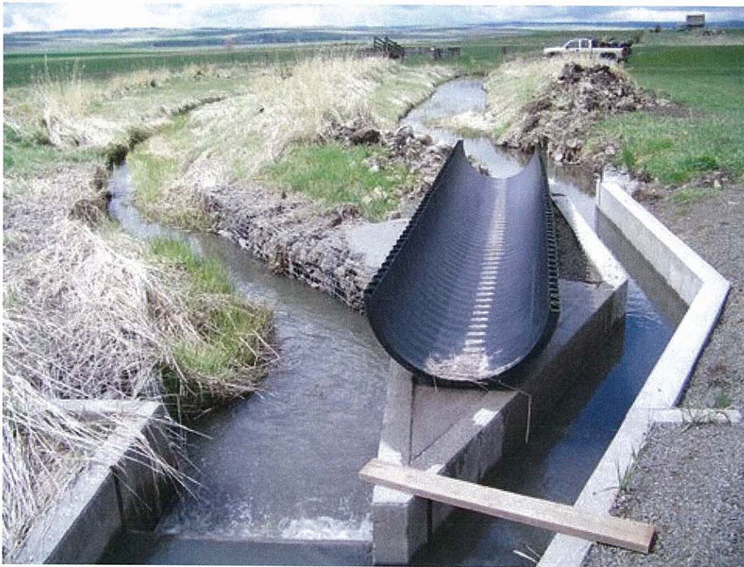
Upstream of diversion looking downstream Spring/Summer 2009. Tolo Lake is located near the tree that can be observed in the far background on the left side of the image.
