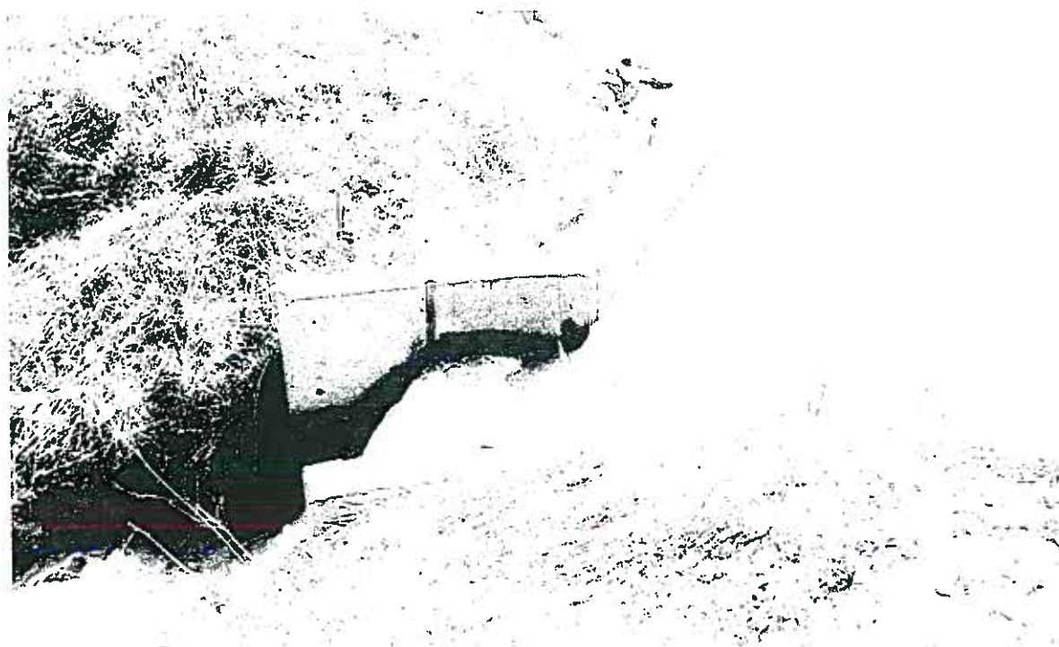
Photo 4: Right (main) spillway, located at right abutment of dam. Note erosion of channel directly below concrete structure.
