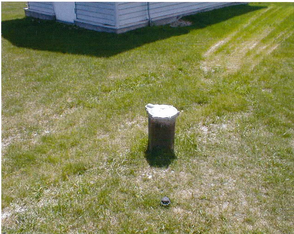
Picture No. 2; East well head, seal, and tag.
