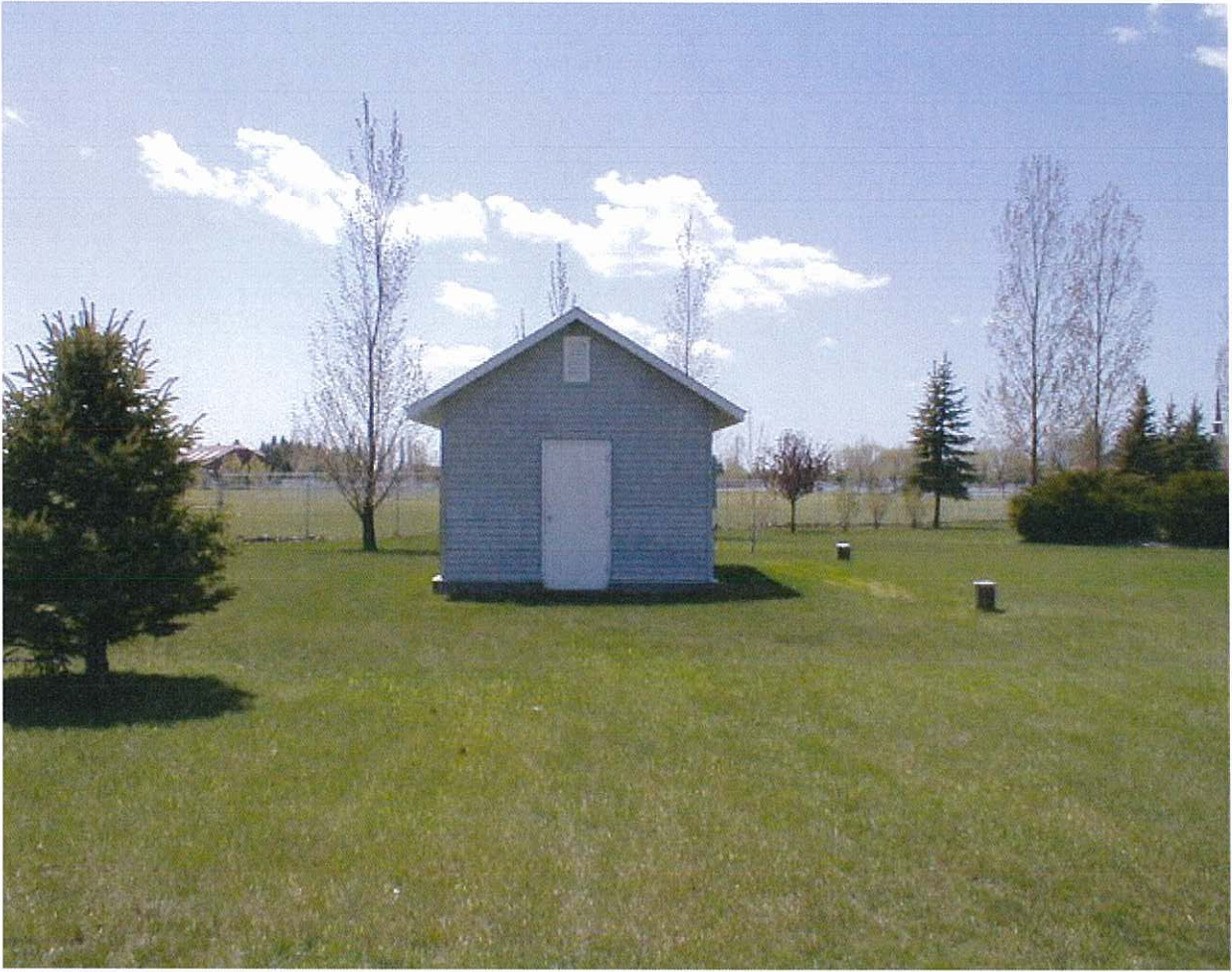
Picture No. 1; Exterior of the utility shed housing pressure tanks and other components.
