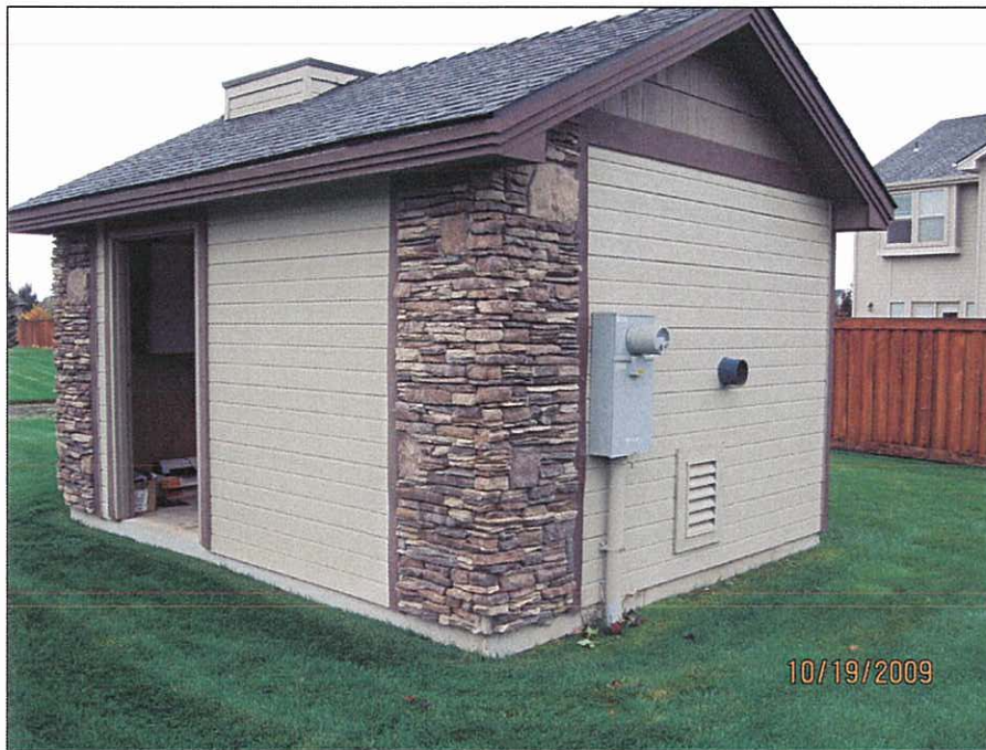
Well pump house
