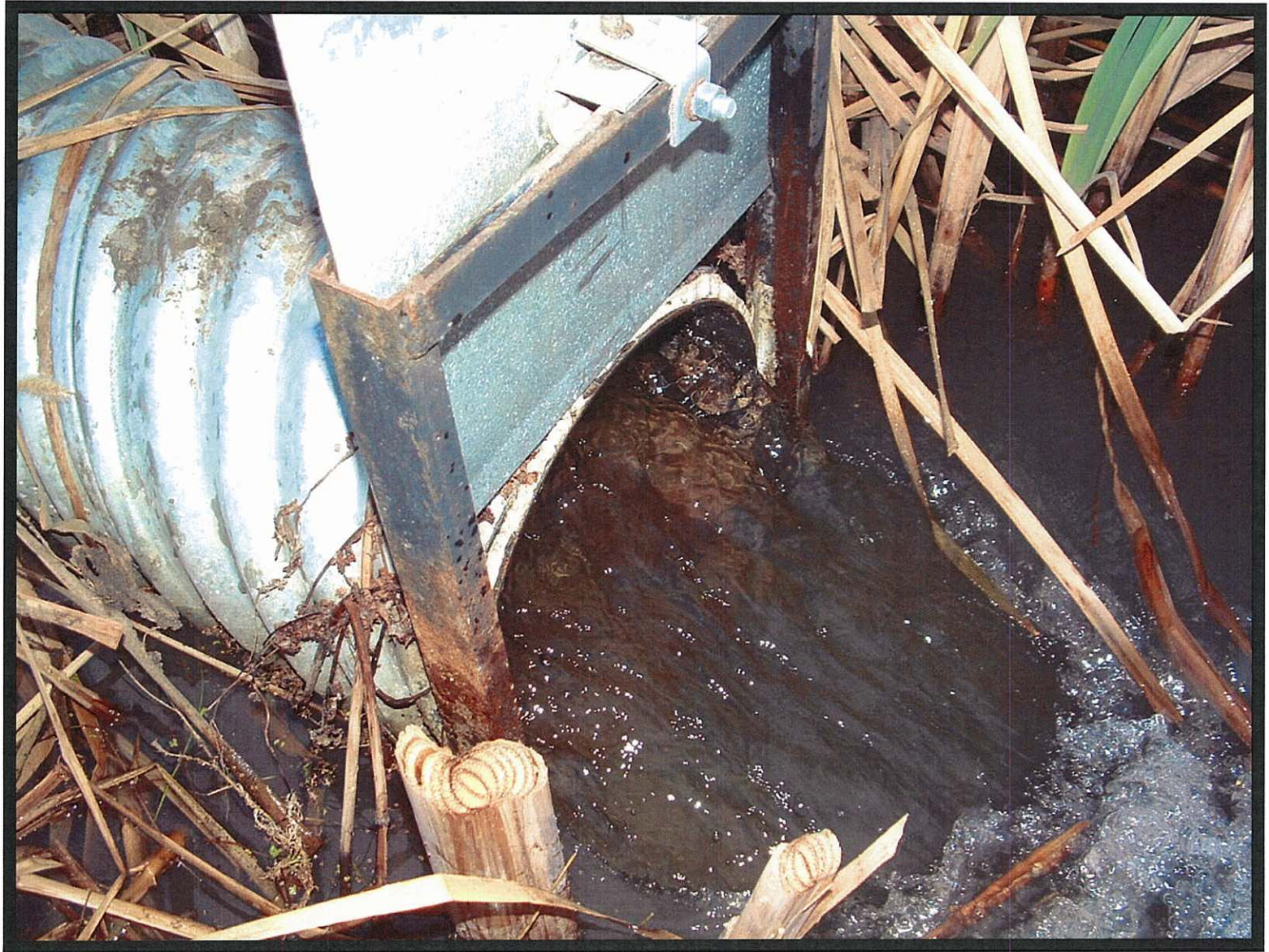
Diversion Works: 12-inch Corrugated Pipe
