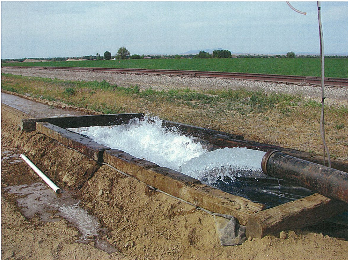
b) Circular orifice weir used to measure flow during stepped-discharge testing of Town Ranch, LP Well #2
