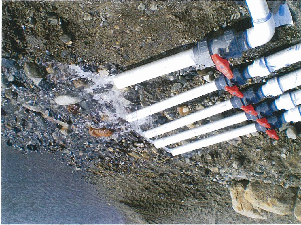
Return to pond for snowmelt Zones 2, 4A, 4B, 4C
