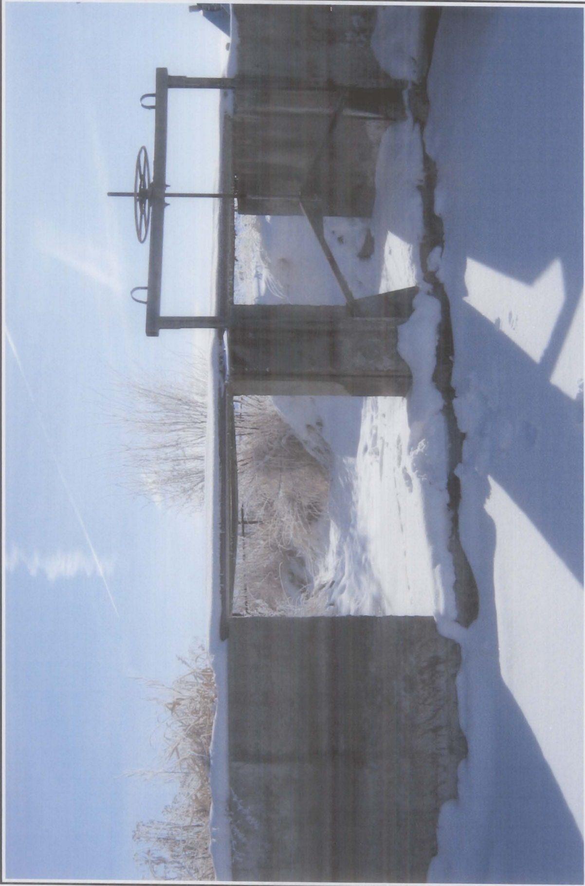
FIGURE 6: SURFACE WATER DIVERSION GATES OFF OF IRRIGATION DISTRIBUTION POND PERMIT NOS. 37-20653 AND 37-20654 THOMAS M. O'GARA FAMILY TRUST
