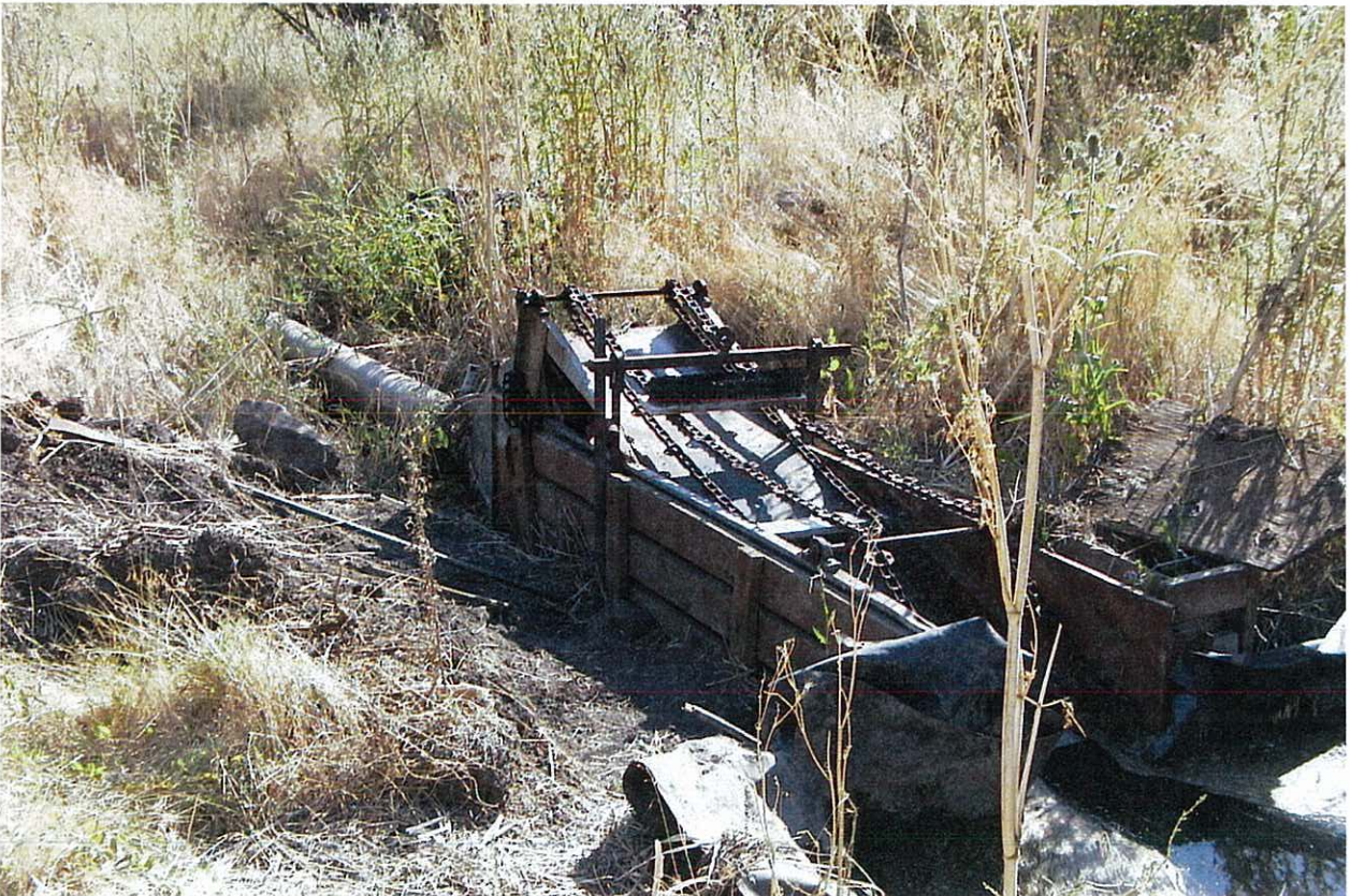
Figure 2: Inactive sluice gate and 12"-diameter pipeline.
