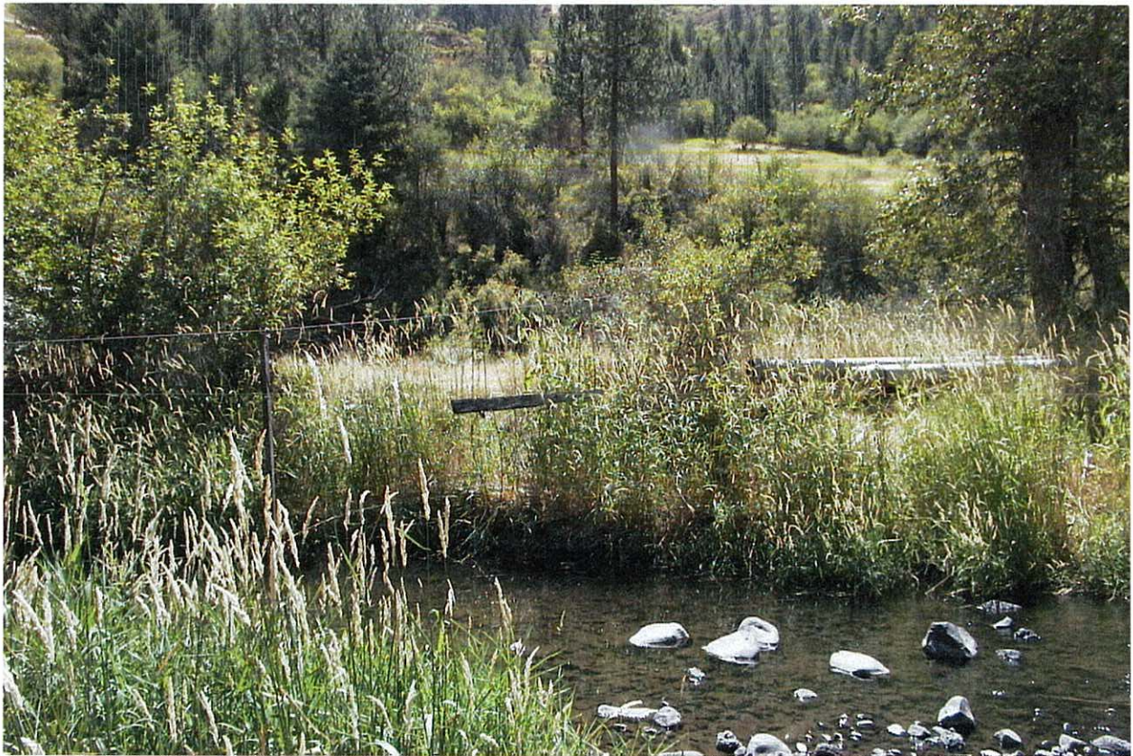
Figure 3: Location of former pipeline-crossing at Lawyer Creek via suspension cable system.
