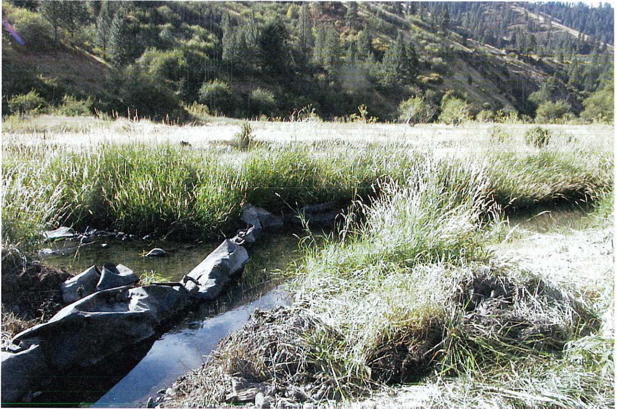
Figure 1: Point of diversion from Lawyer Creek, earth and tarp diversion dam.
