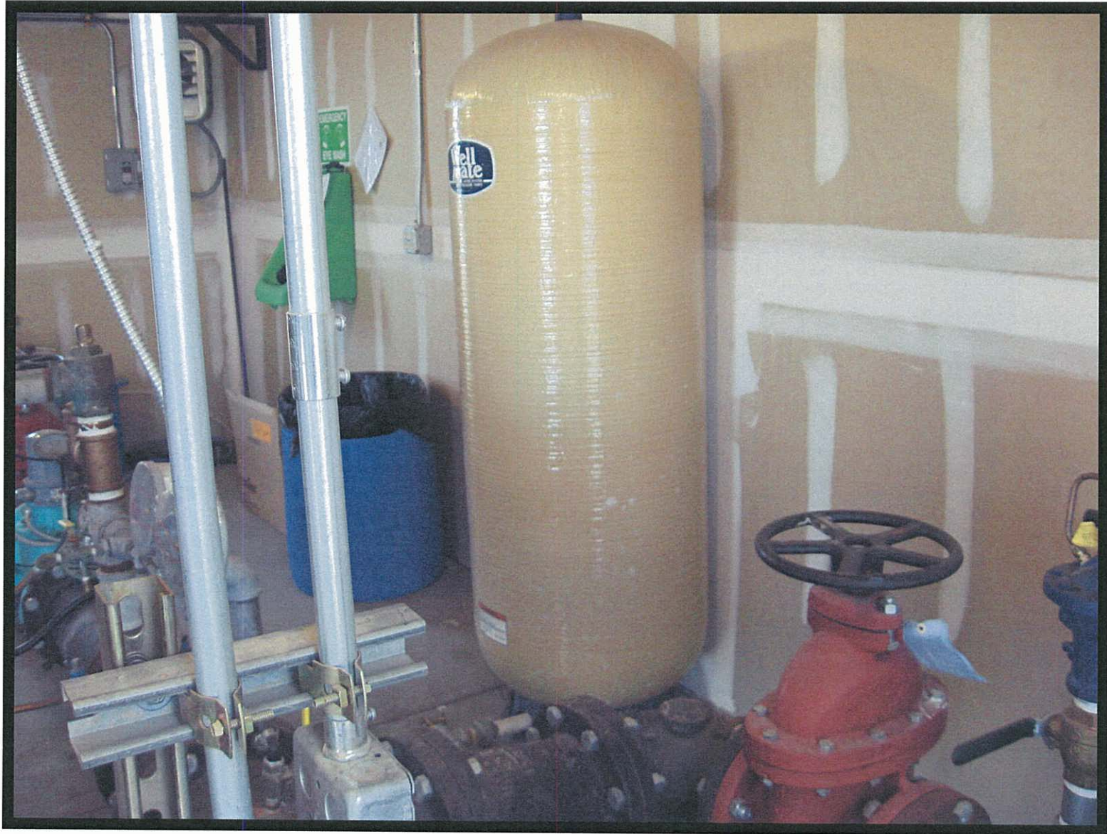
Hydropneumatic Tank
