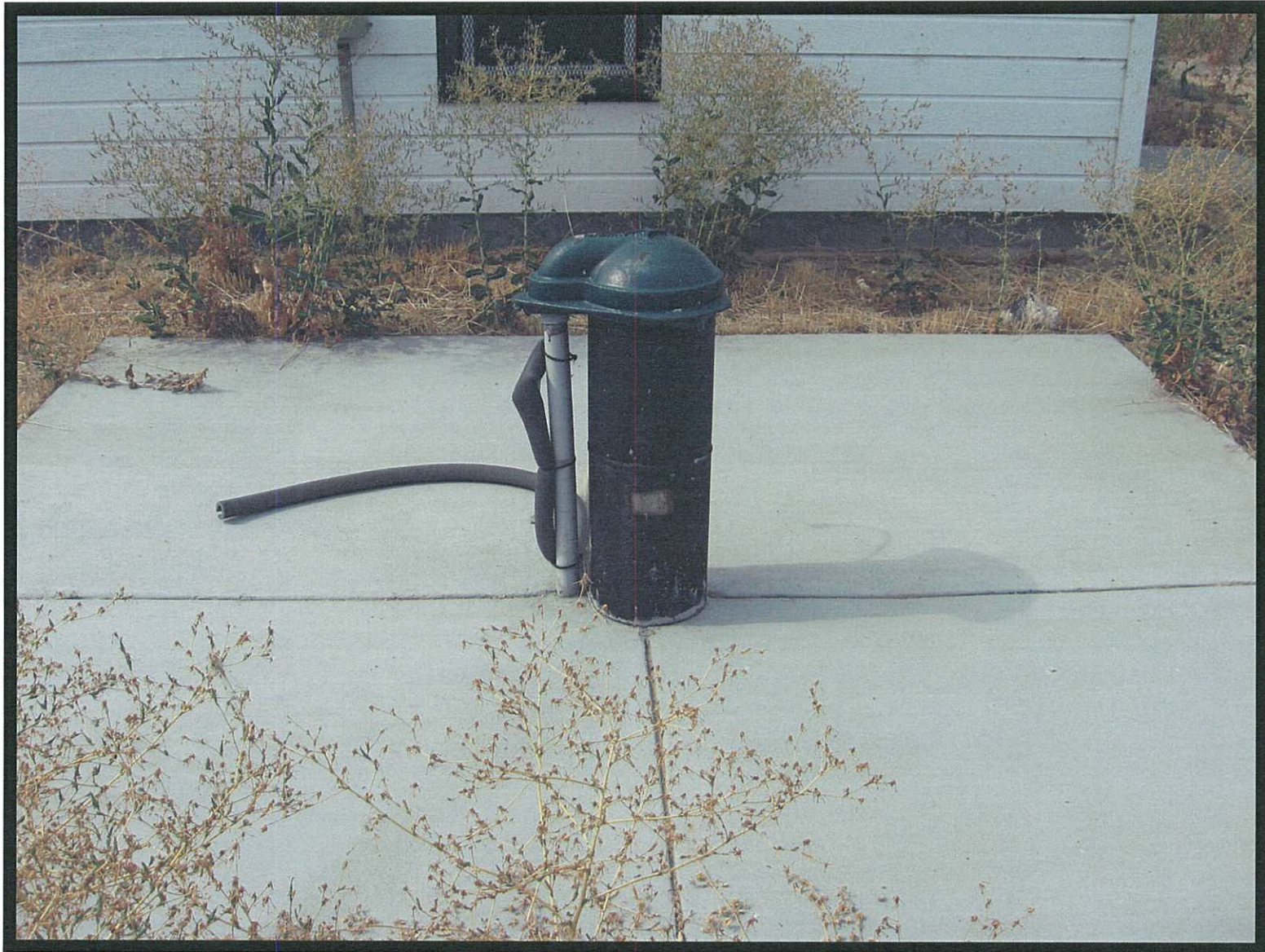
Well No. 1 (Primary Well)
