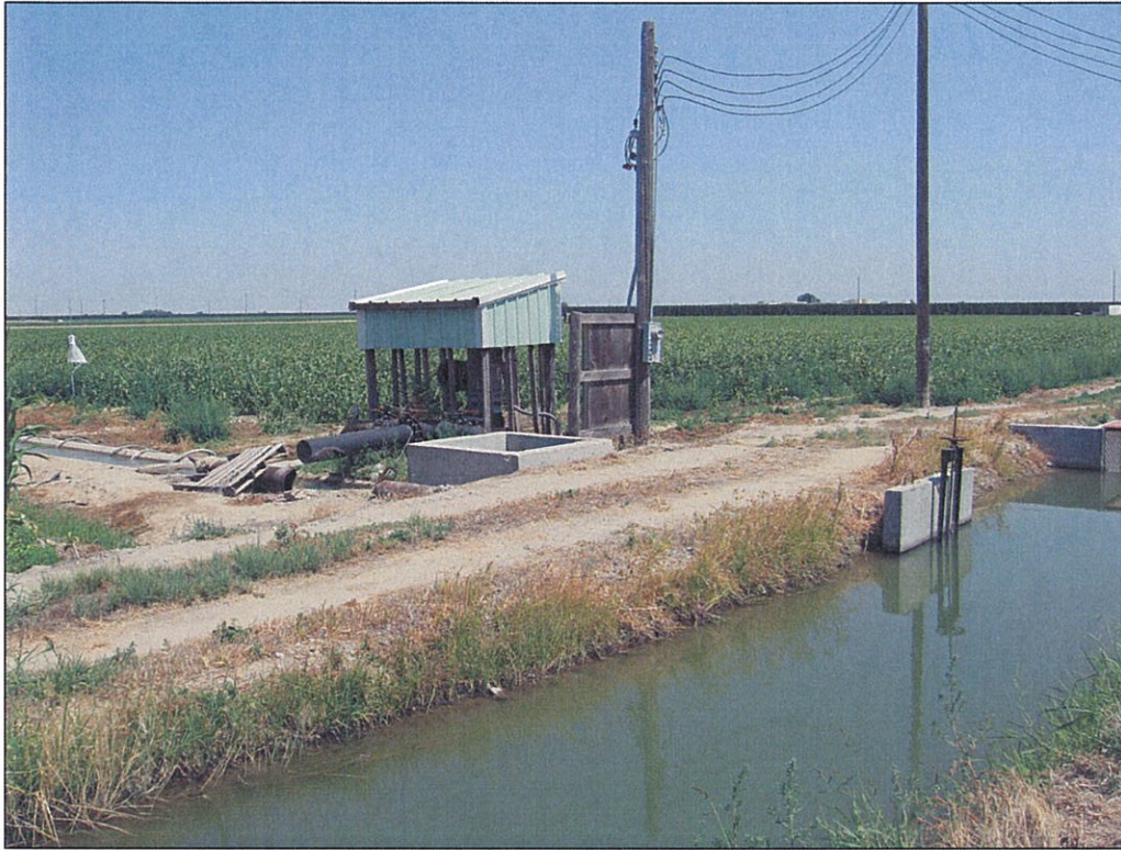
Figure 3: Well, facing northeast. Paine Lateral in foreground.
