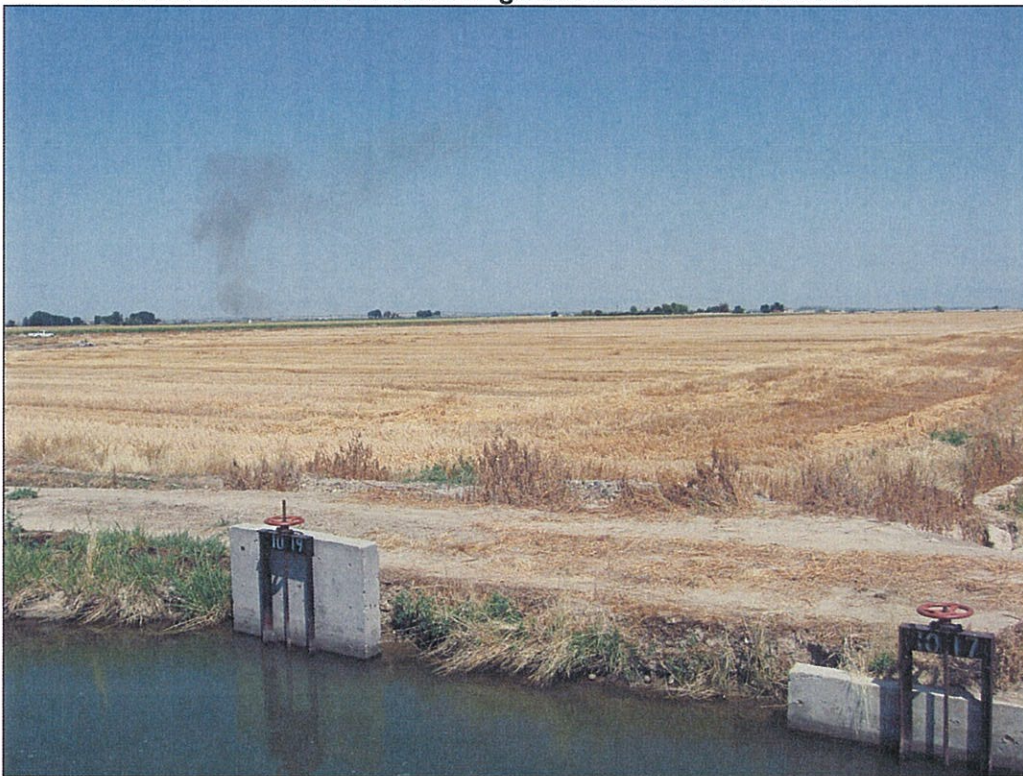
Figure 12: Photo taken at the southwest corner of NWSW Section 12, facing northeast. Turnouts 1017 (right, closed) and 1019 (left, open) from the Drew Lateral serve the S1/2 and the N1/2 (respectively) of the N1/2 of the SW 1/4 Section 12. Turnout 1017 serves the harvested grain field shown in this photo.
