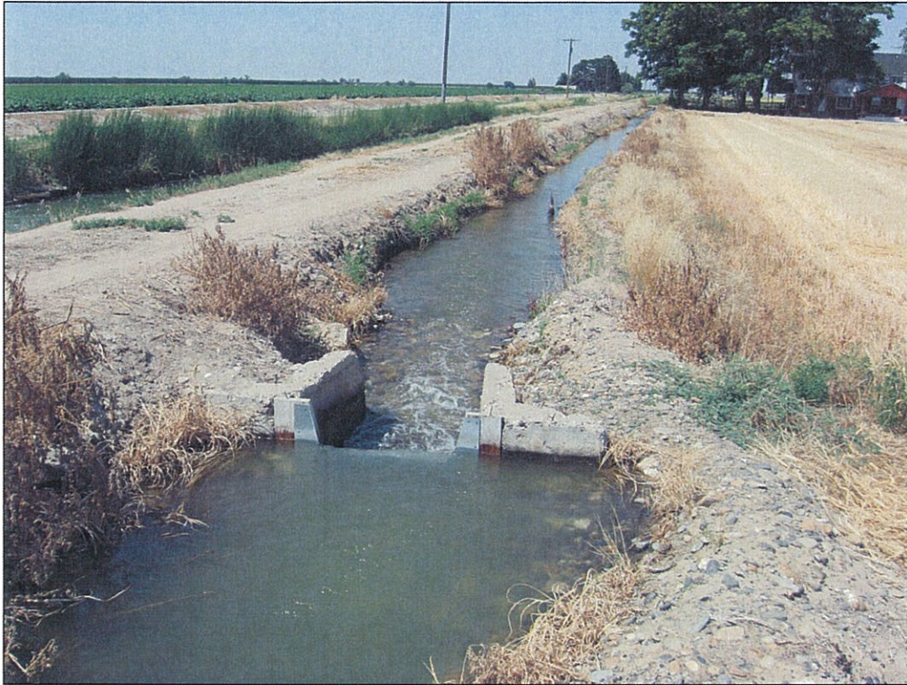
Figure 13: Photo taken near turnout 1019 showing flow diverted by this turnout from the Drew Lateral and serving N1/2 N1/2 SW1/4 Section 12 (corn field beyond trees and home in background on right)
