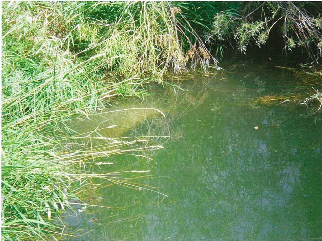
Outlet of 36" reinforced concrete pipe
