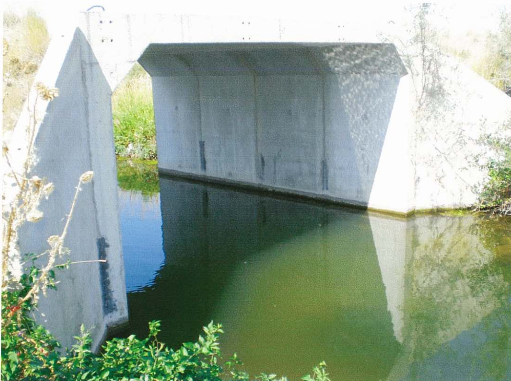
Upstream side of box culvert bridge – measuring point
