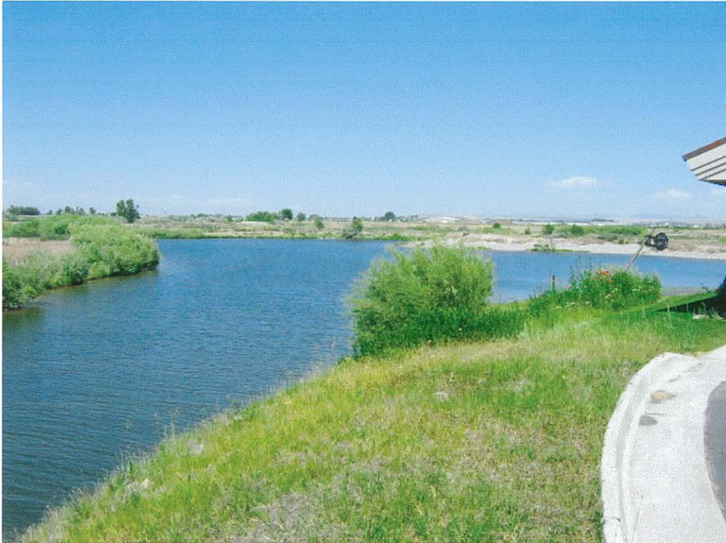
Gem Lake Harbor looking northeast from return point
