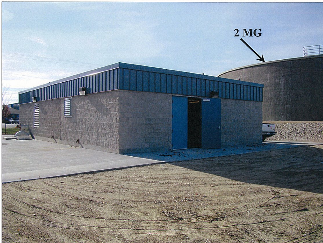
b) Photo looking southwest at Well #20-B side of pump house with 2 million gallon tank in background.
