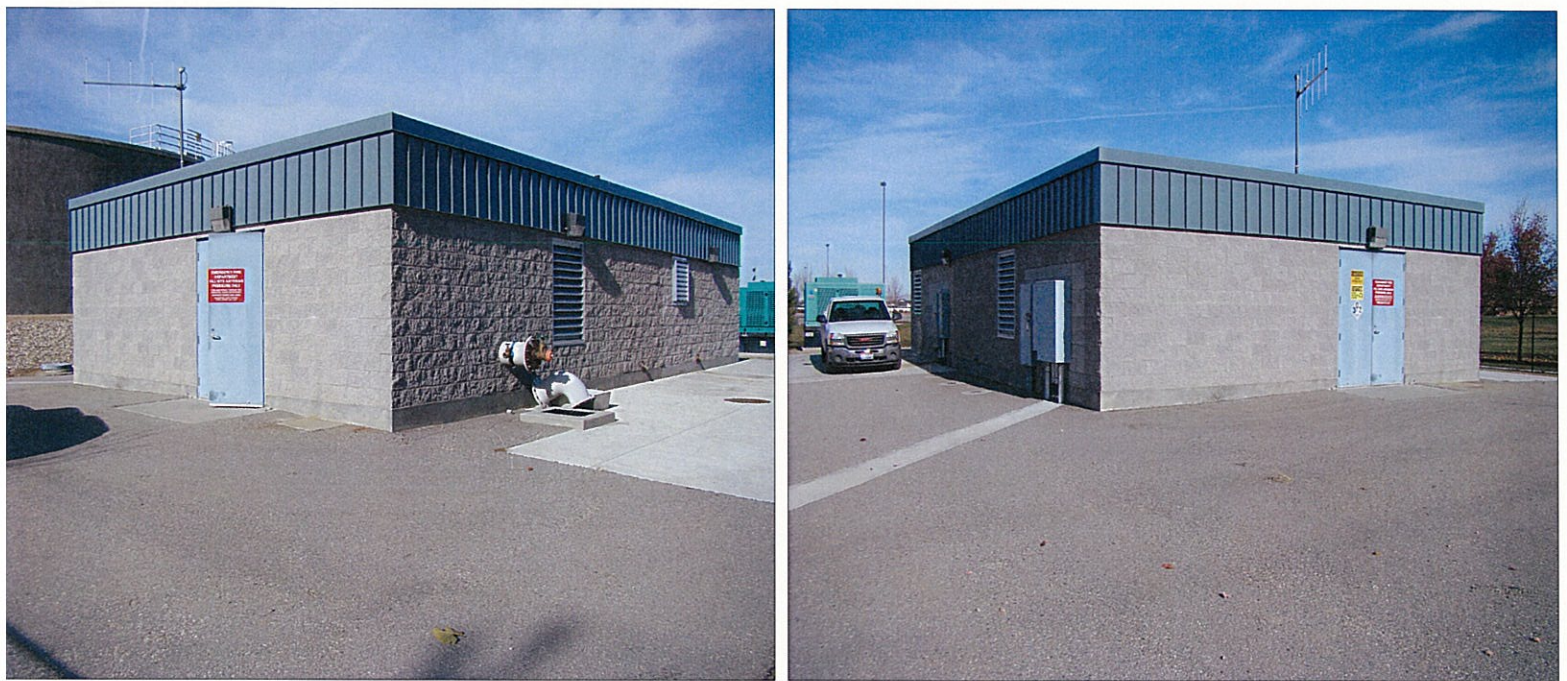
a) Views looking at Well #20-A side of pump house. (looking NW on the left and NE on the right)
