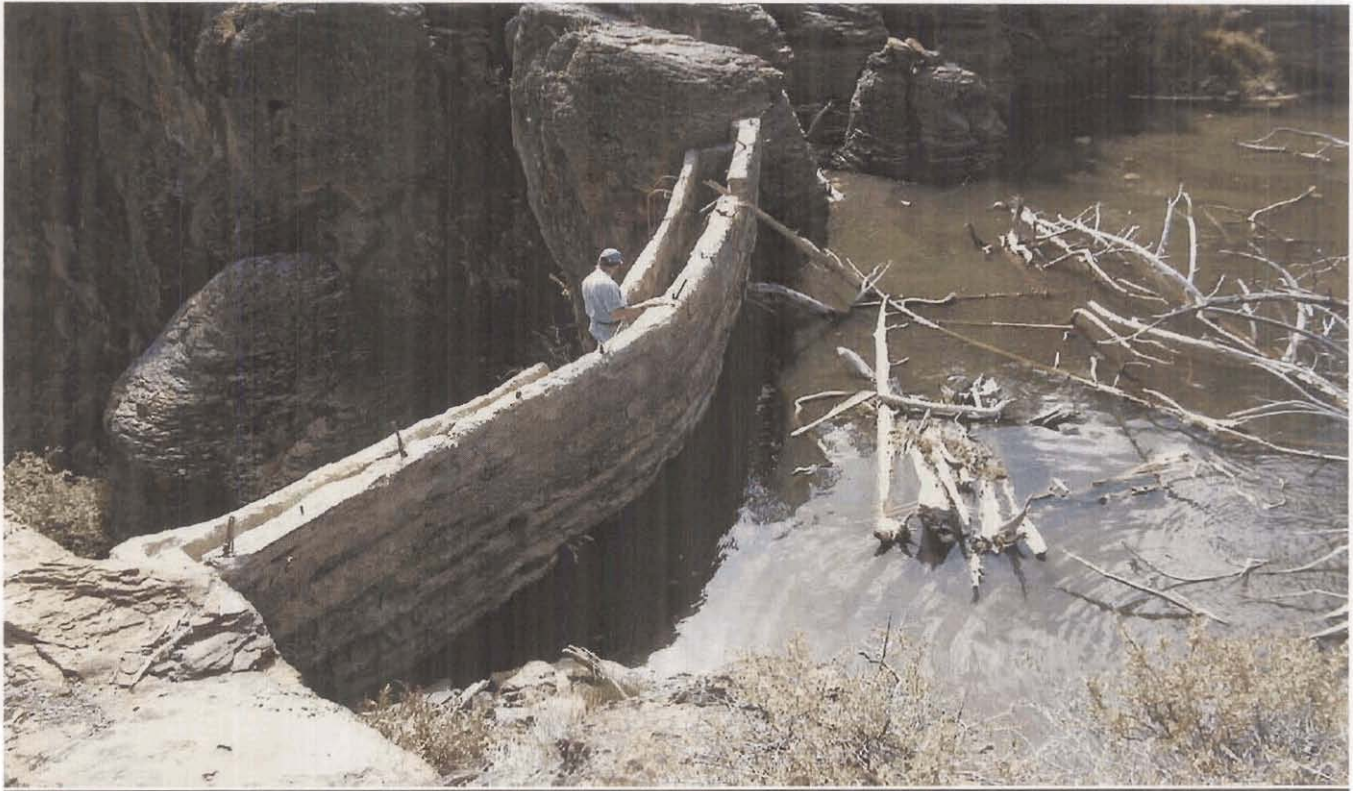
Photo #1: Dam upstream face.
