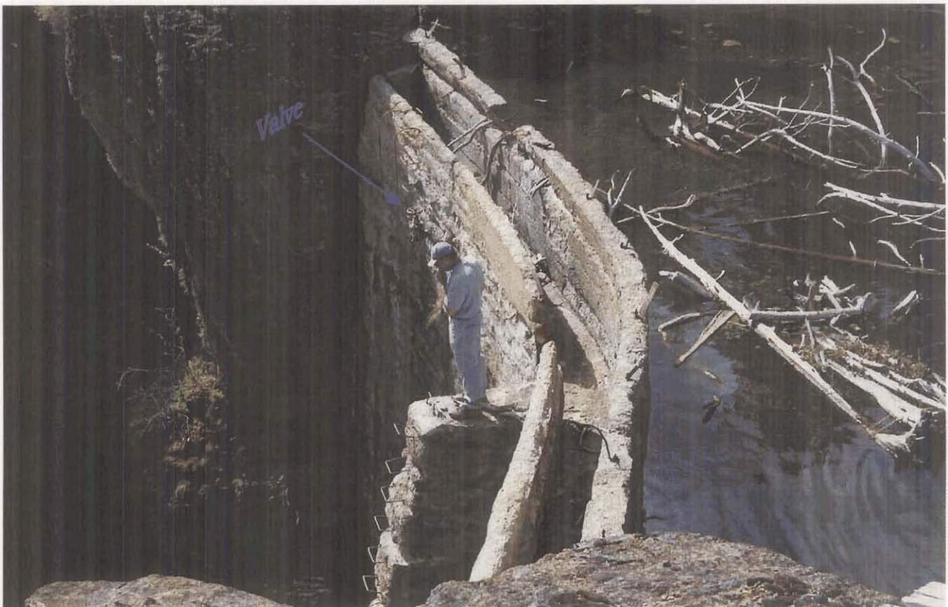
Photo #2: Overview of the crest parapet wall
