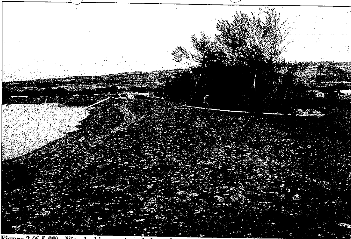
Figure 2 (6-5-09) - View looking westward along the northern side of the dam, taken from near the diversion ditch. The portable pump is discharging water from the reservoir into Grossen Creek.
