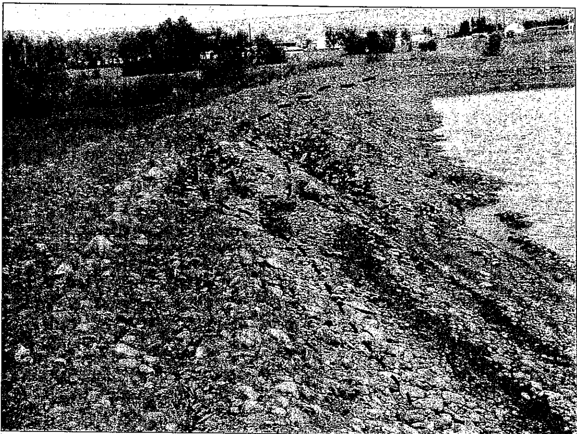
Photo 1 (6-5-09) - View looking north along the western, centerline axis of the existing embankment dam. The pool level is approximately 4 feet lower than first observed yesterday when it was within just a few inches from overtopping the dam, as indicated by dashed line. At its narrowest dimension, the dam crest is only about 6 feet wide. Construction materials were obtained from the pool area and pushed up to create the perimeter embankment. The dam was built without IDWR dam safety approval; neither was it designed by a licensed professional engineer.
