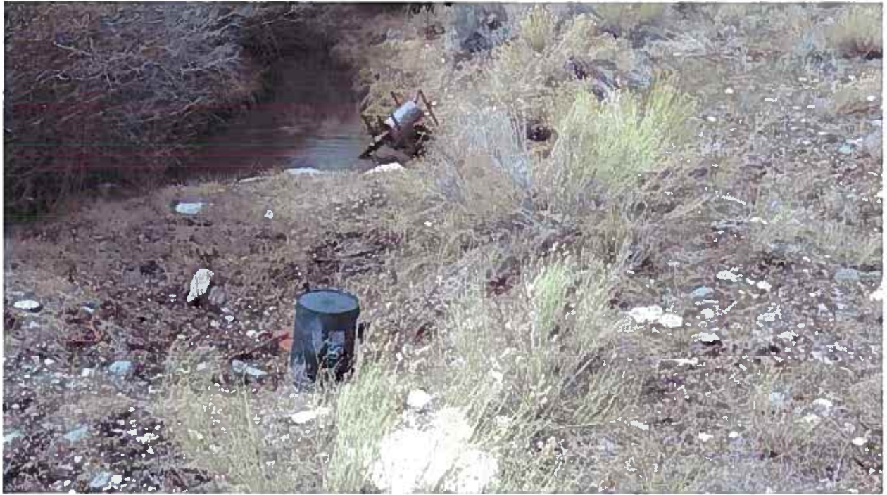
Photo 5 View looking upstream of the Entire Diversion system
