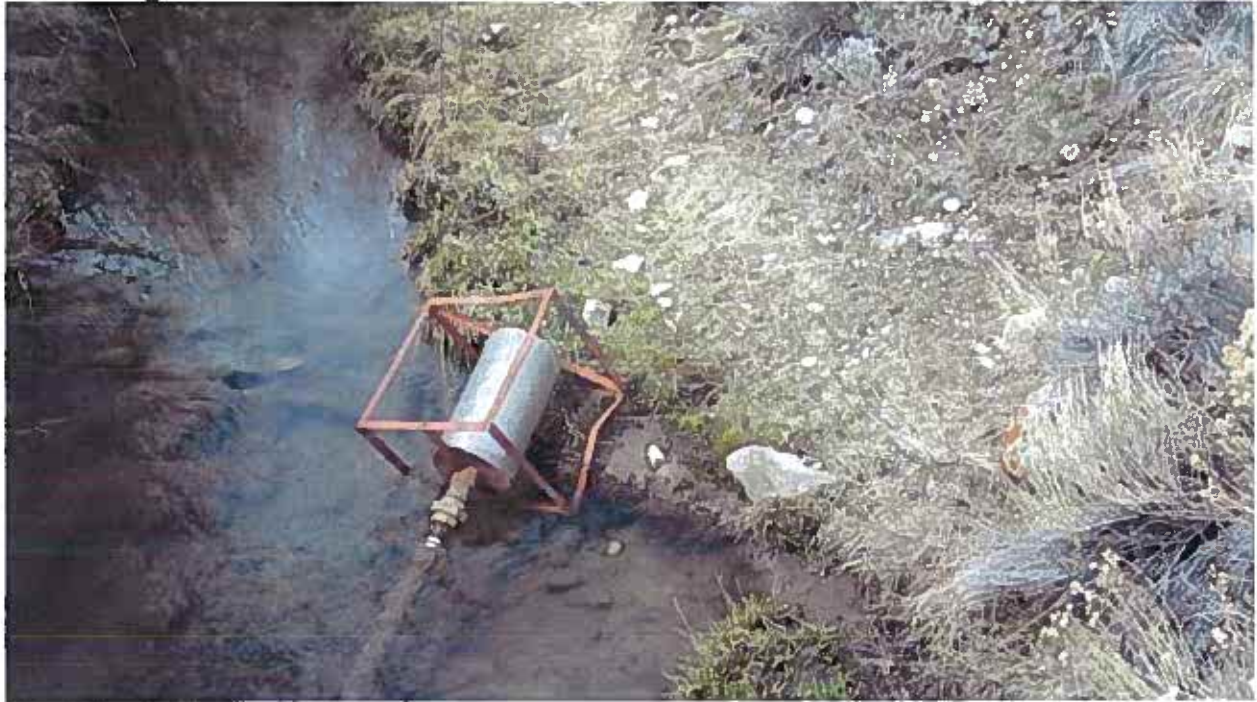
Photo 1 The diversion structure looking upstream
