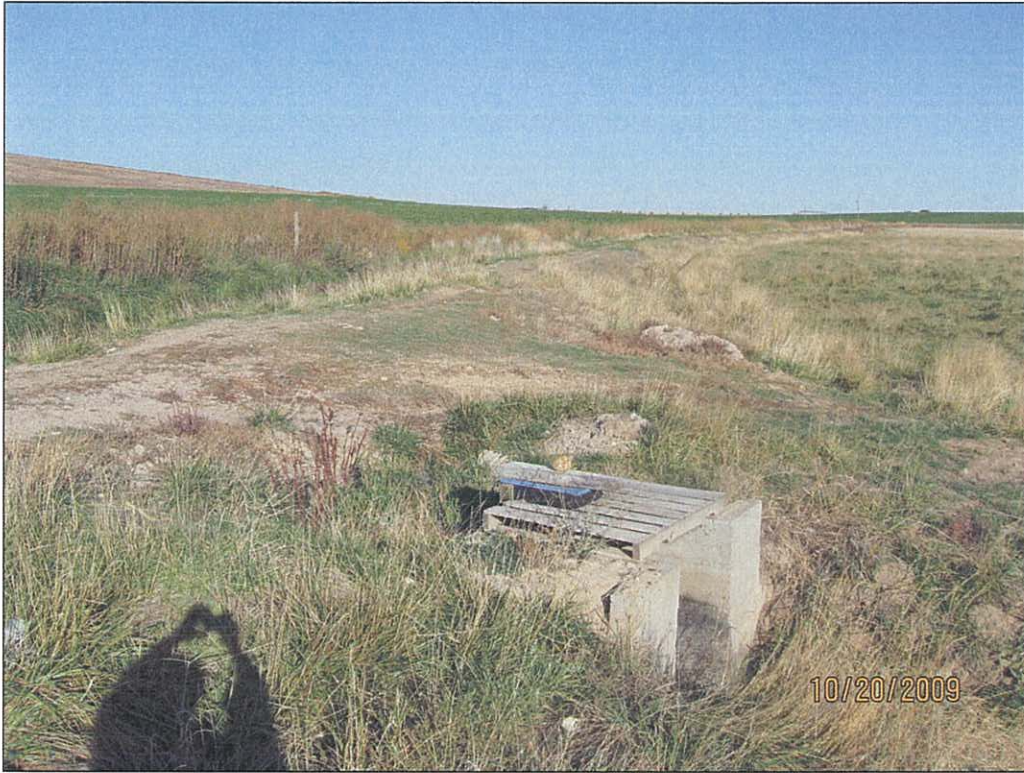
Photo 3: Upper "Turnout #1" from Hat Butte Lateral with well pump in far right background.
