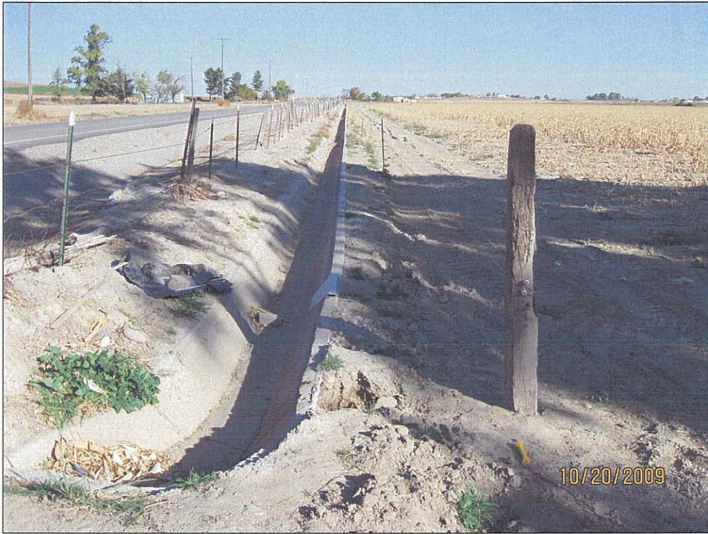
Photo 9: Southwest corner of irrigated place of use facing north.
