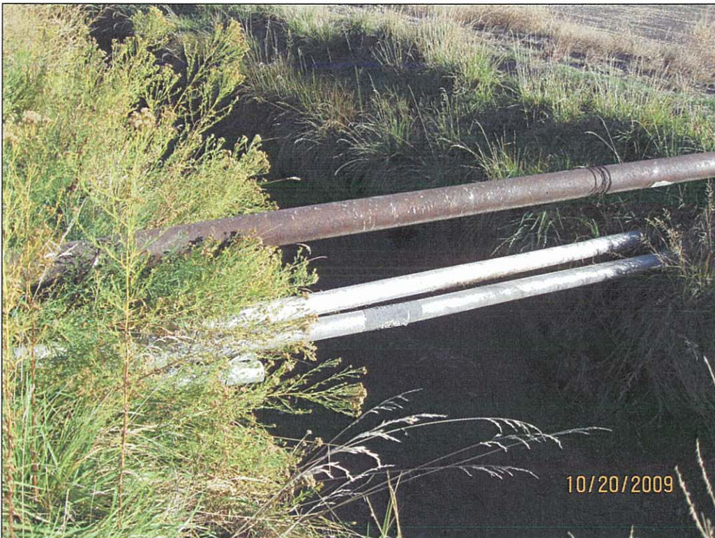
Photo 2: Aluminum pipe discharges into Hat Butte Lateral about 40-feet east of well pump.
