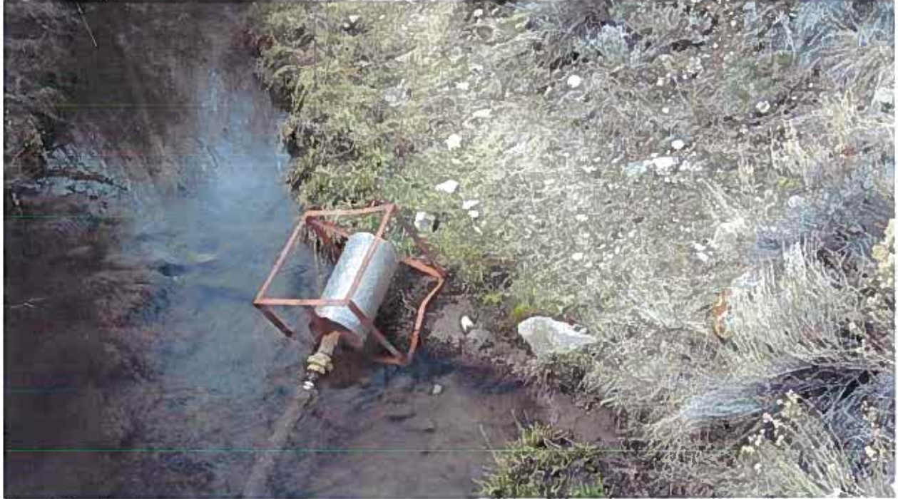
Photo 1 The diversion structure looking upstream
