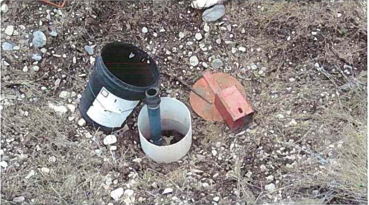
Photo 3 Overflow Pipe at POD
