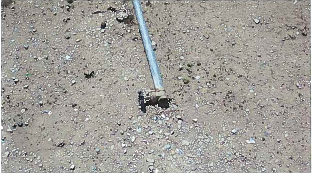
Photo 13 Valve at the end of the Troughs
