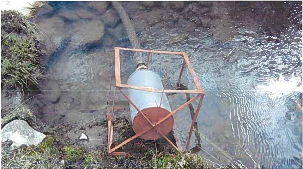
Photo 2 The diversion Structure looking downstream
